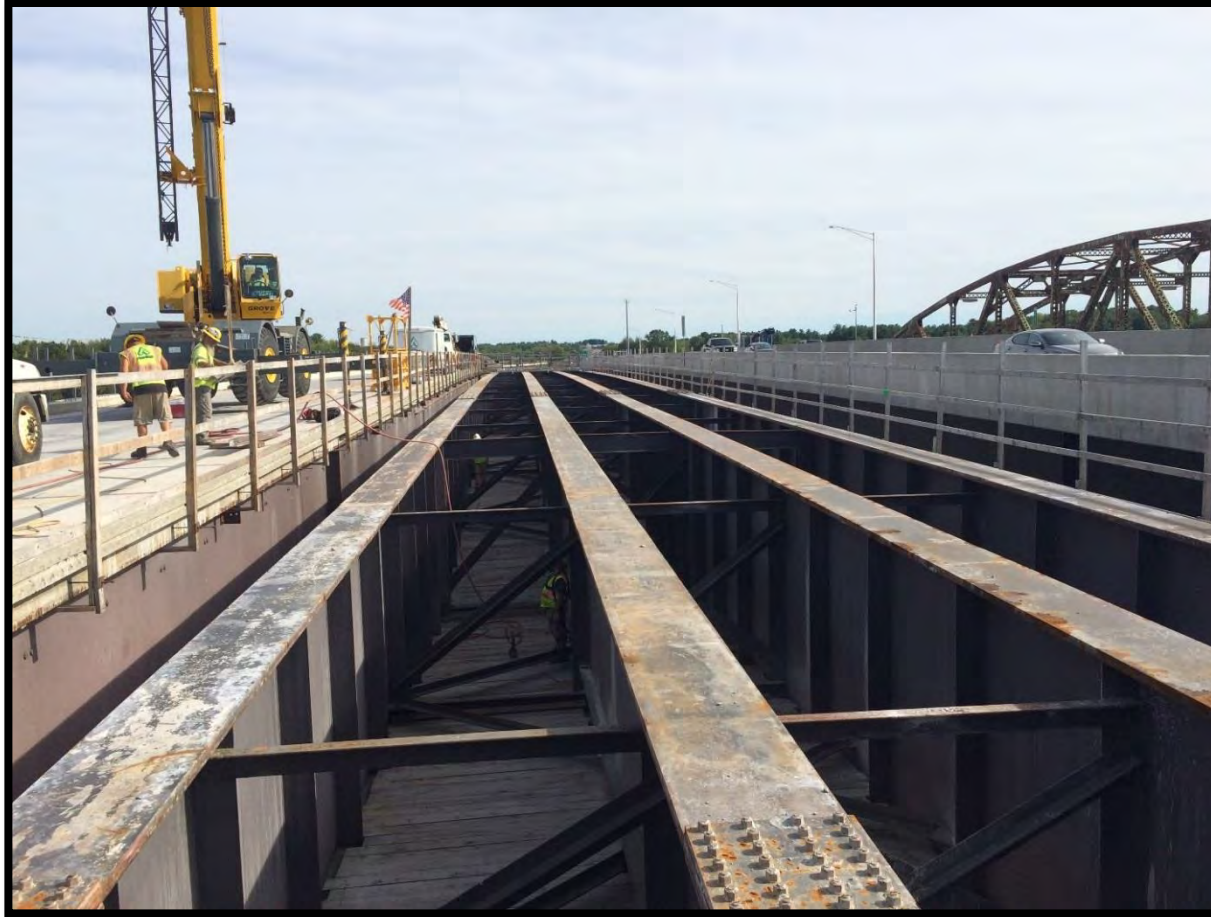
Bridge Girders Following Concrete Deck Removal
