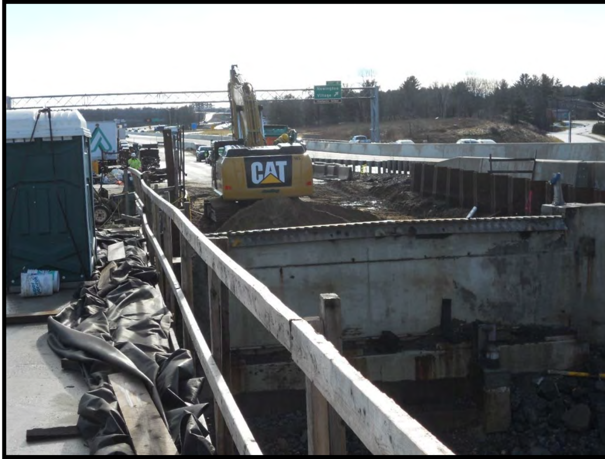
Bridge Abutment Work in Newington
