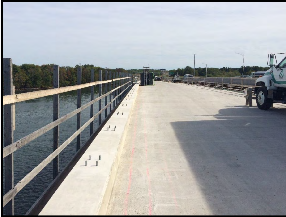
Concrete Bridge Deck with Coping for Bridge Guardrail
