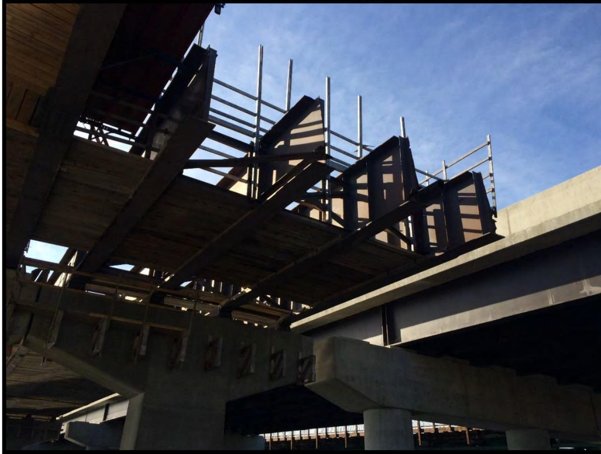
Partial Bridge Girder Removal
