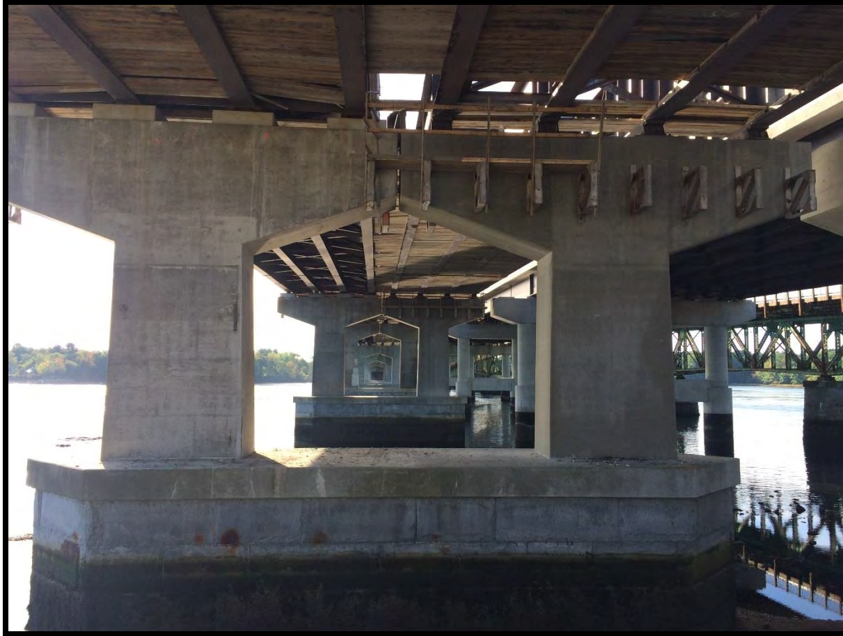
River Piers and the Underside of Bridge
