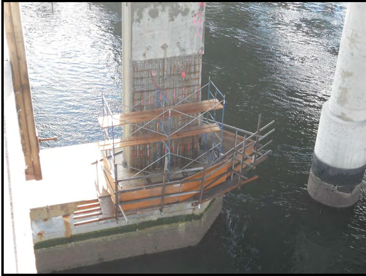
Concrete Pier Rehabilitation
