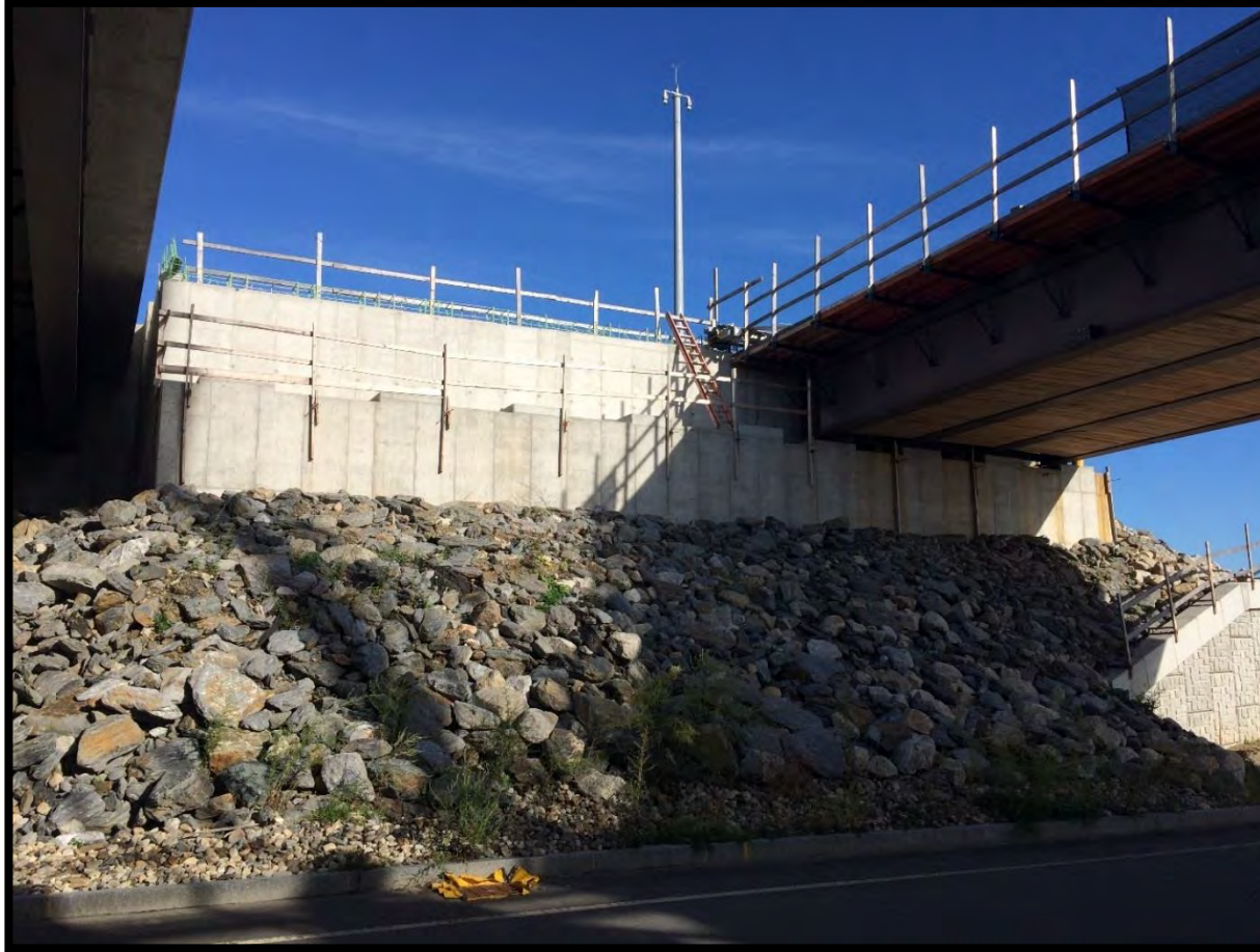
Dover Bridge Abutment from Wentworth Terrace
