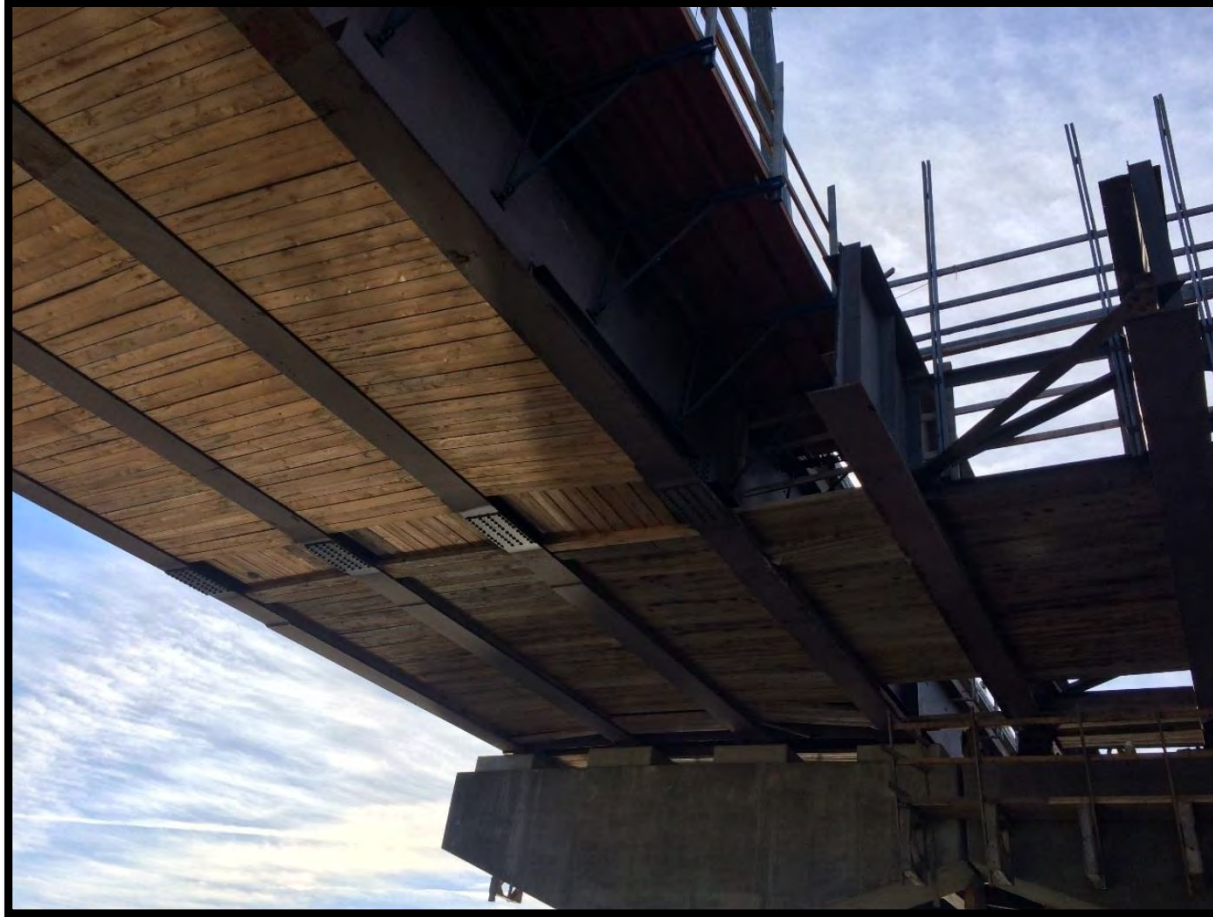
Bridge Girders and Pier on Dover Side
