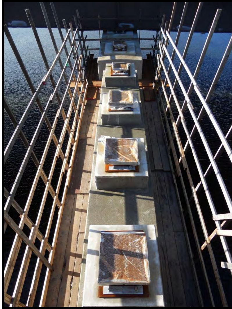
Bridge Pier with New Bridge Seats and Bearings Waiting for New Girders
