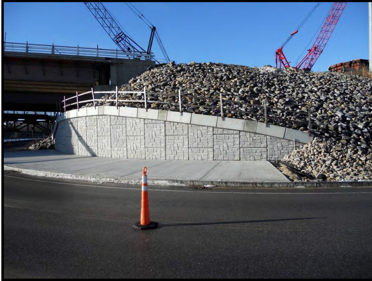
New Retaining Wall Beneath Little Bay Bridge On Wentworth Terrace
