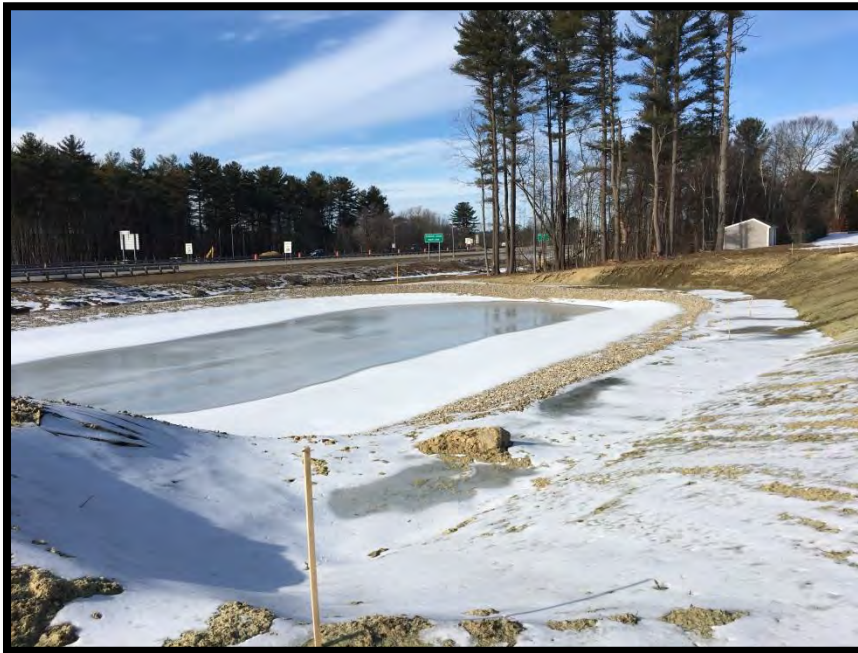
Exit 6W Storage Area
