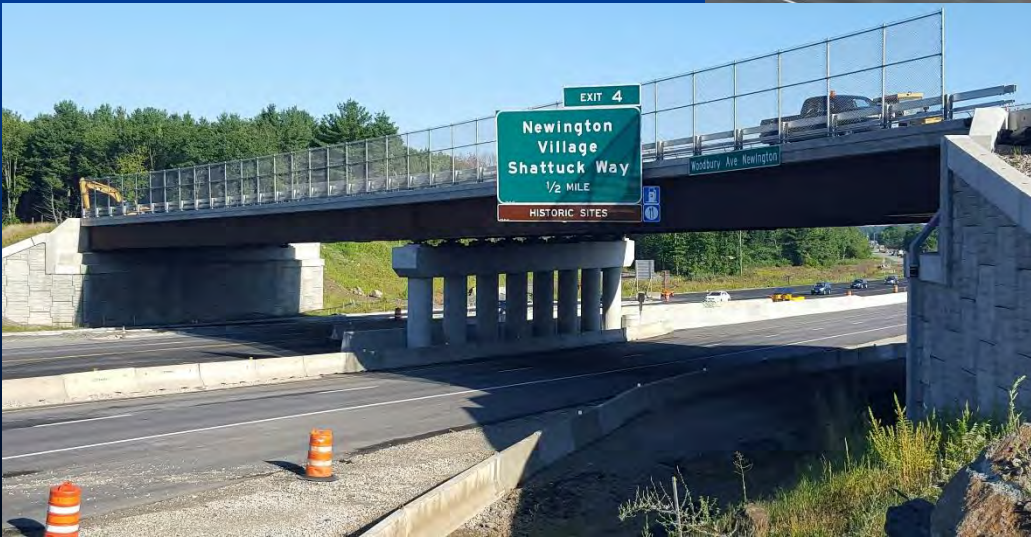
Woodbury Avenue Bridge – looking NB
