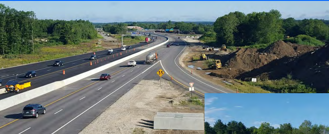
Exit 3 NB On Ramp
