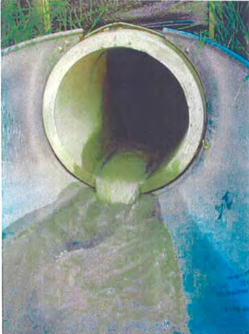
Photo A. Culvert discharging to Great Bay immediately to the east of the Exit 4 underpass to the Spaulding Turnpike. Although only 1" deep (approx, not measured) water is opaque due to sediment and turbidity from DOT construction sites west of the turnpike.
