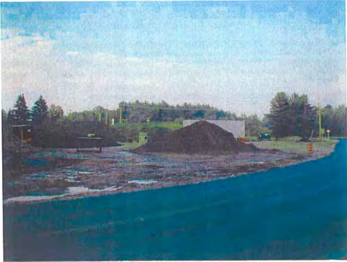
Photo B. Looking Southeast towards Nimble Hill Road from Exit 4. No erosion controls or swales present. Storm drain is located adjacent to the road near the standing water. Water containing sediments is washing off the site directly on to the road or into the storm drain.
