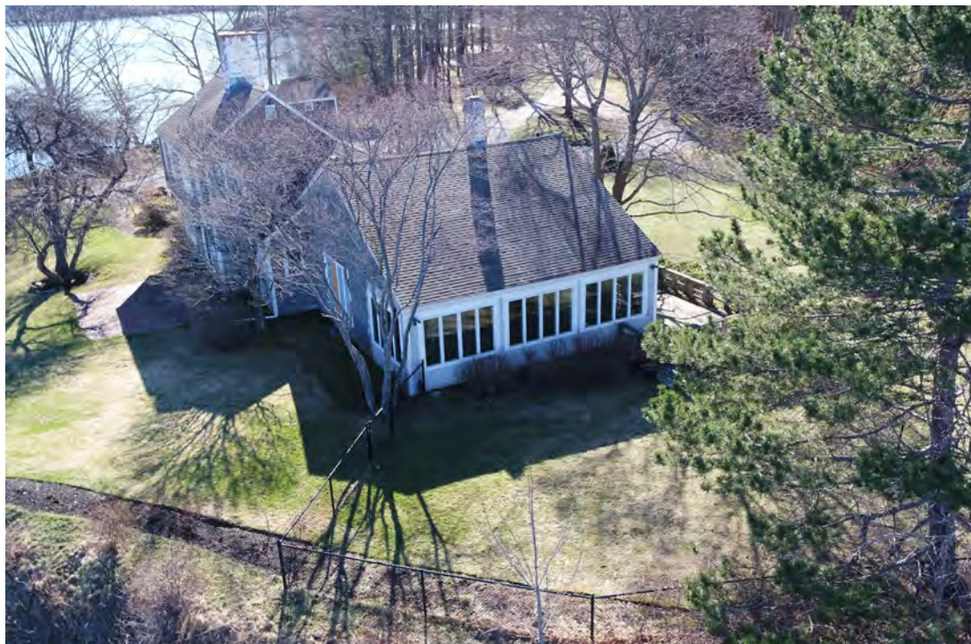
Photo # 5 Description: 137 Beane Lane, rear (north) and west elevations with west addition in foreground Reference (file name or frame #): NWN0246_5 Direction: E Date: May 2019
