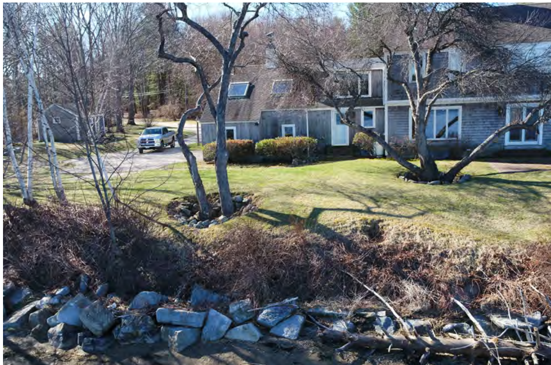
Photo # 2 Description: 137 Beane Lane, rear (north) elevation of east addition (left) and main block (right)
