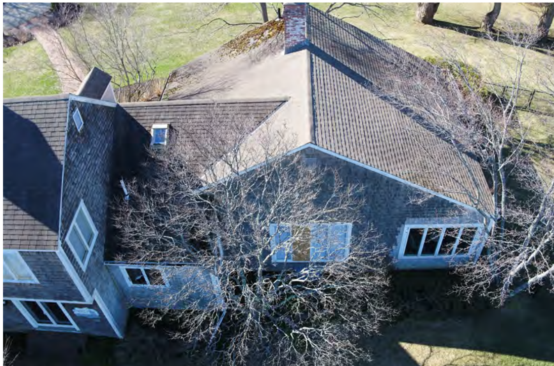
Photo # 4 Description: 137 Beane Lane, rear (north) elevation of west addition Reference (file name or frame #): NWN0246_4 Direction: S Date: May 2019
