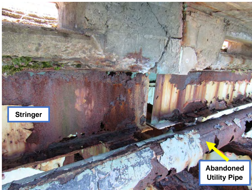
Photo D9: Span 7 and 8 Stringer at Deck Joint
