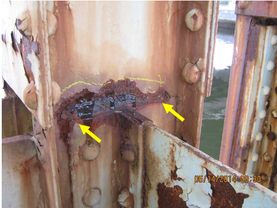
Photo D32: 2014 Inspection – Span 7 East Member L8U8
