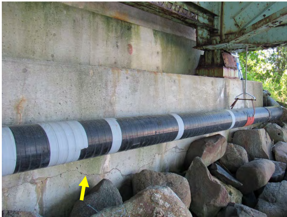
Photo D44: Newington Abutment – Horizontal Crack in Breastwall
