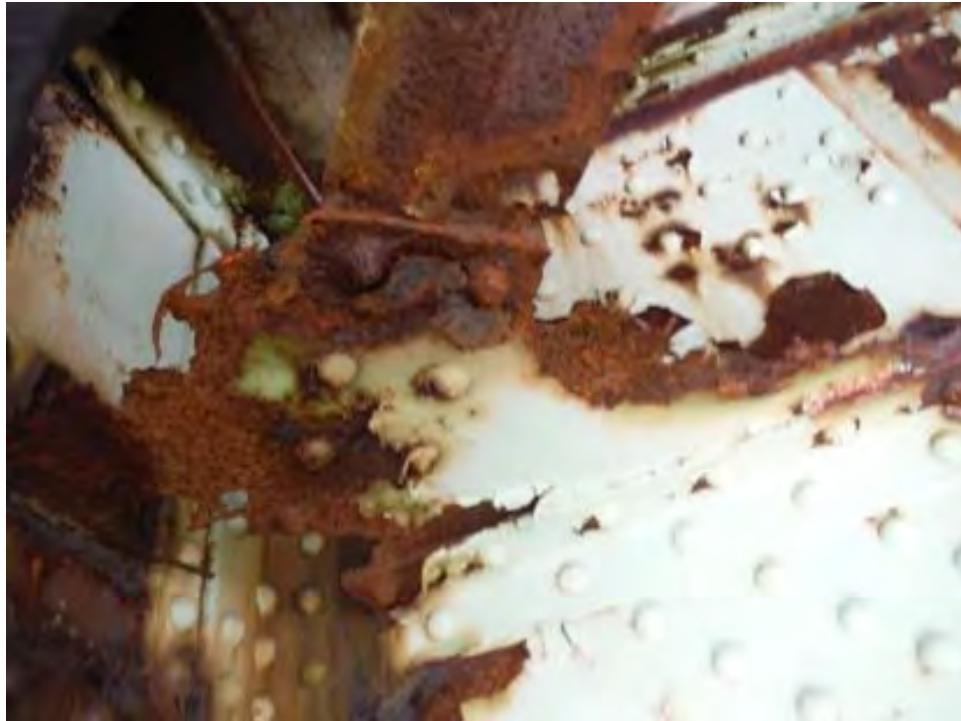
Photo B.5: Span 4, lateral gusset plate U1. Severe section loss in lateral gusset plate, with 100% section loss in connection to floorbeam. Many severe cases exist throughout Spans 4, 5 and 6.
