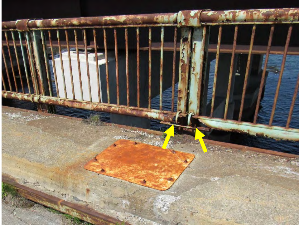
Photo D3: Span 3 East Bridge Railing – Lower Rail Section Loss
