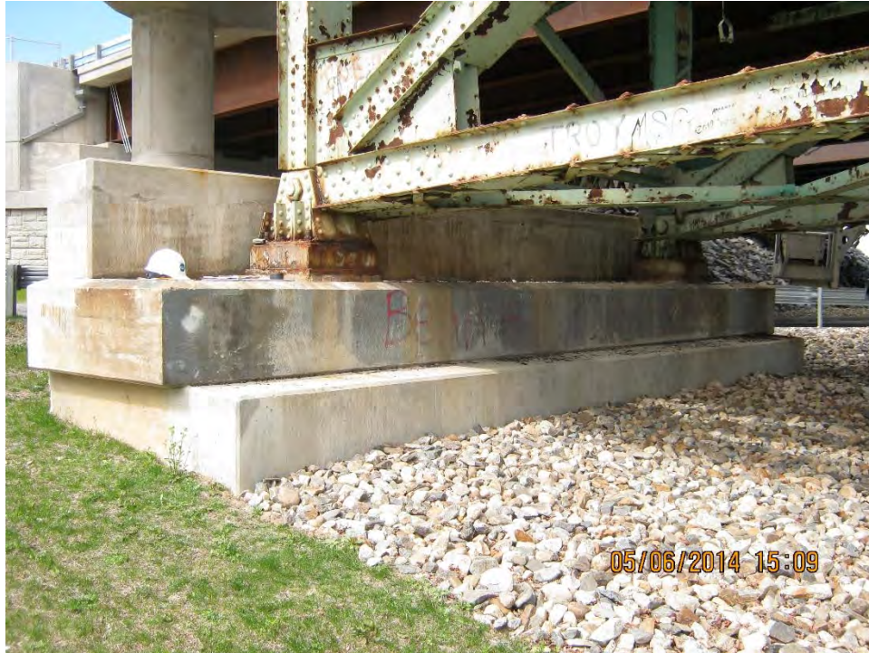
Photo S.1: Dover abutment in overall good condition.
