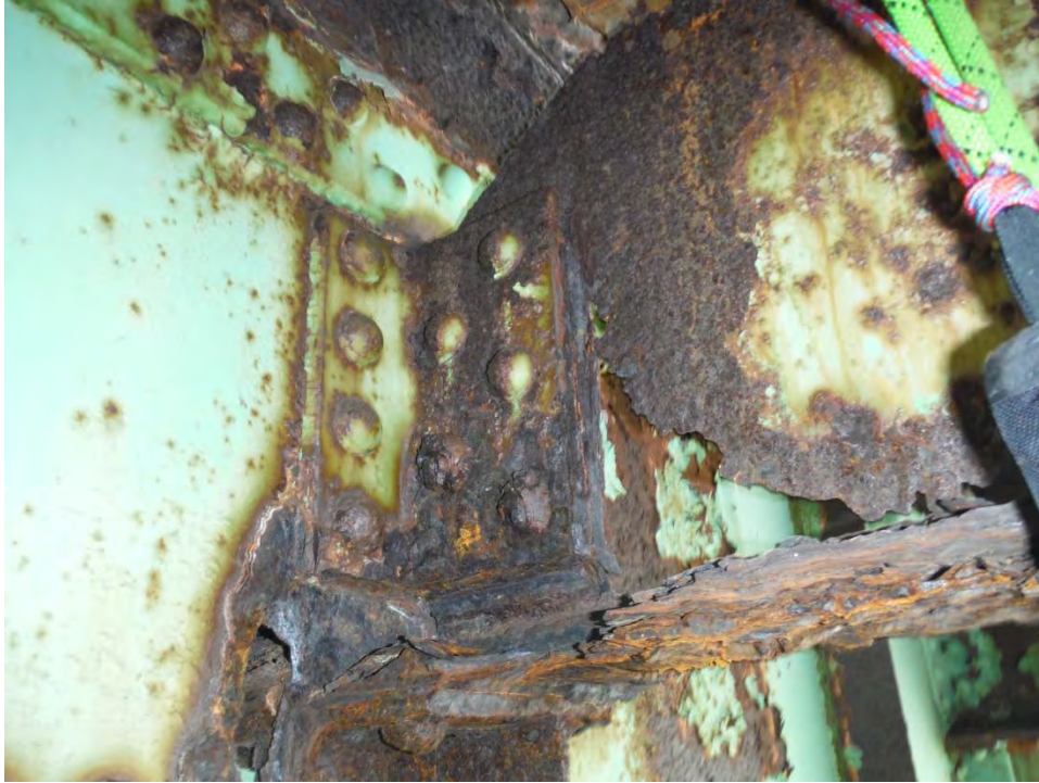
Photo F.9: Span 6, east stringer connection at Floorbeam 7'. Corrosion holes and section loss in web of stringer and in floorbeam.
