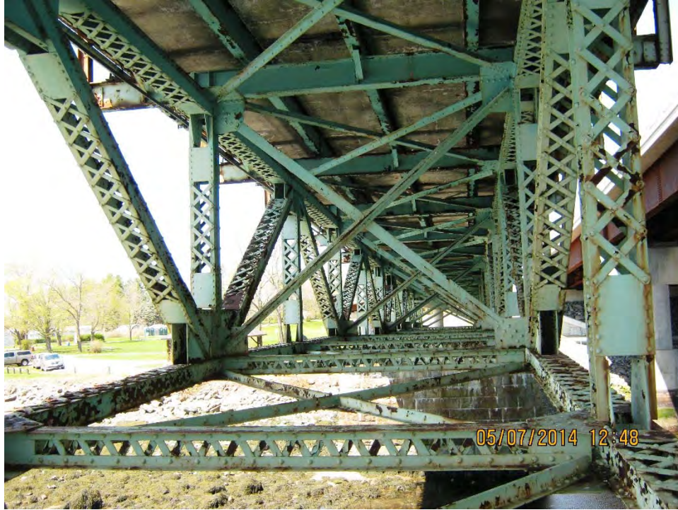
Photo: T.3: Span 2, built-up channel members throughout the truss generally in fair to poor condition.
