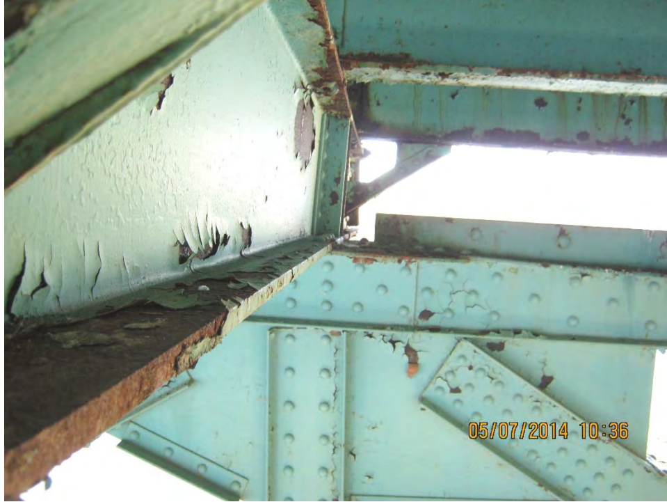
Photo F.11: Span 2, floorbeam F1. All floorbeams in Span 2 are racked 5°- 10° to the north. Similar conditions exist on Span 9 floorbeams.
