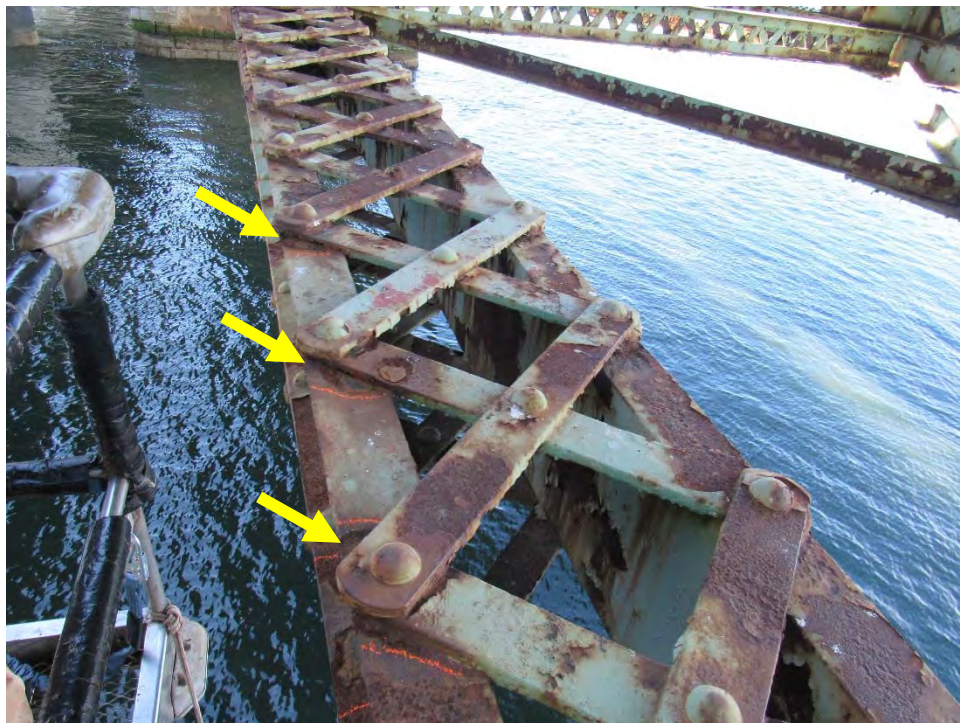
Photo D21: Span 3 Bottom Chord – Section Losses at Lace Bars
