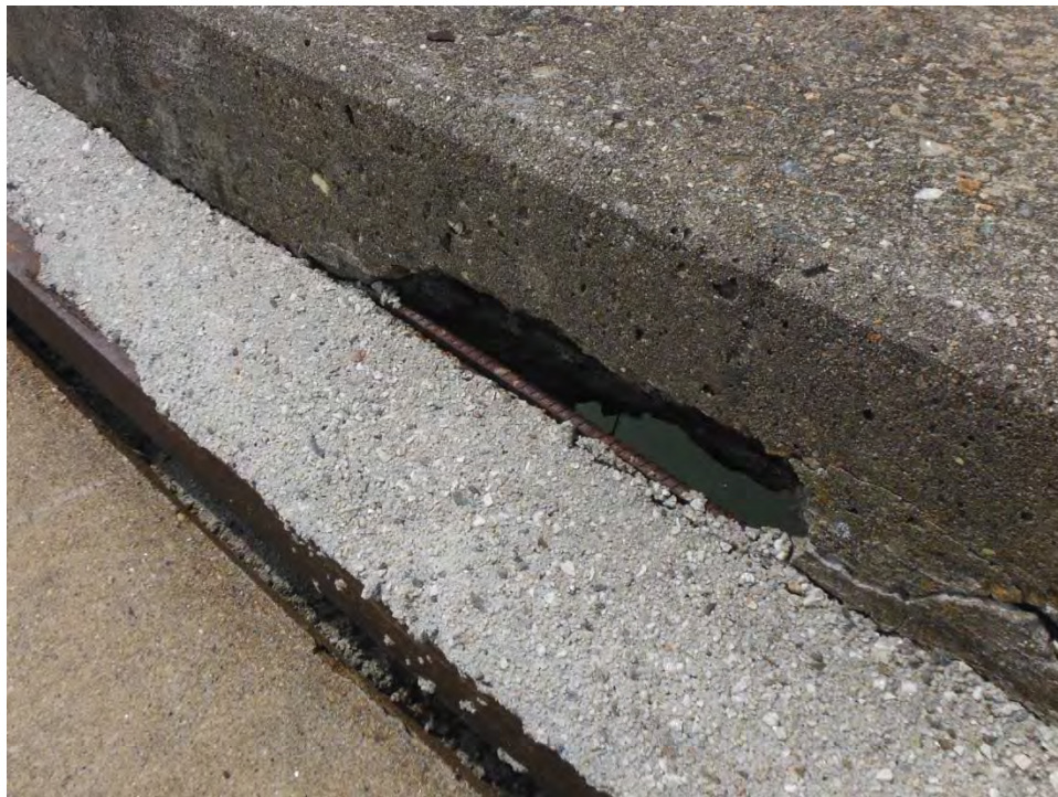
Photo D.6: Span 6, west curb at mid-span. Spalling and cracking in curb at mid-span. Stringer at this location exhibits signs of overstress
