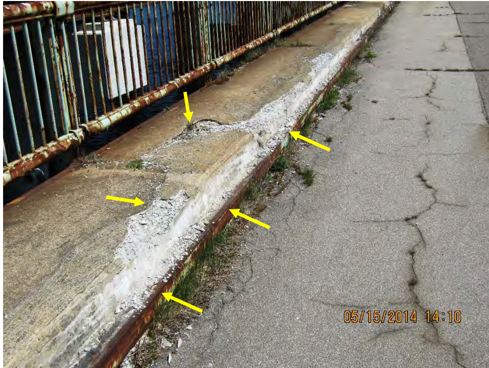
Photo D.5: Span 1, curb over east fascia. Large area of curb spall where channel has separated from curb and large cracks have formed. Similar condition exists on several locations throughout the deck.
