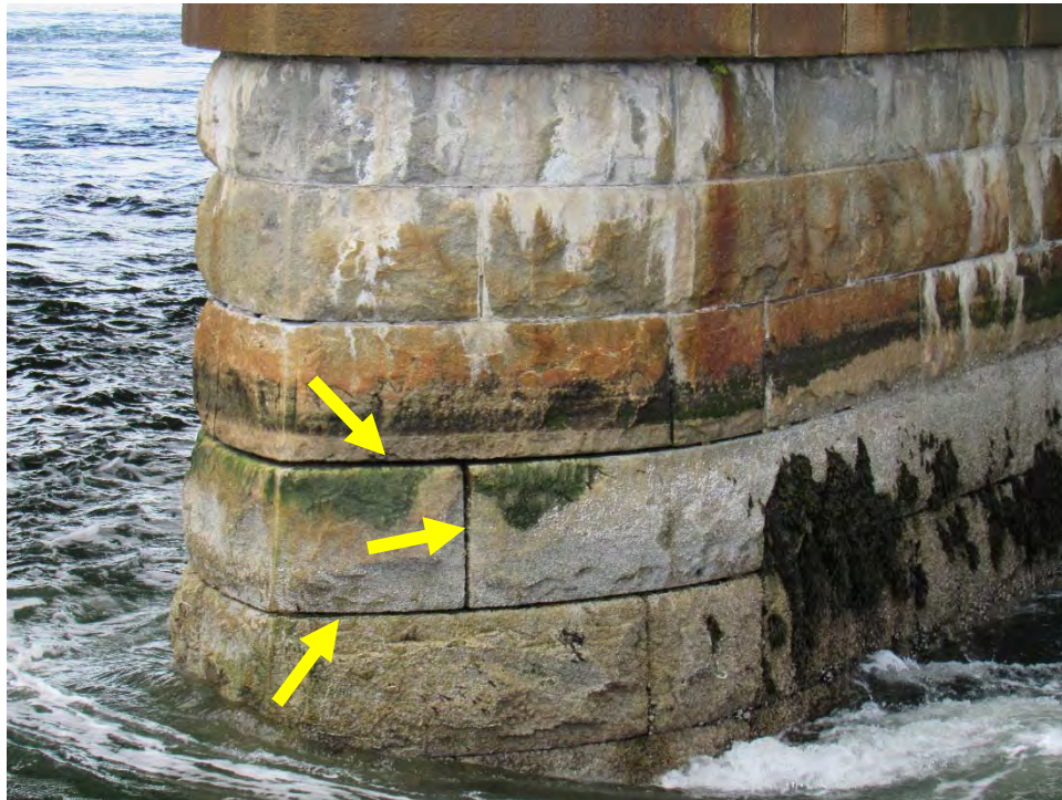
Photo D45: Pier 7 – Missing pointing mortar
