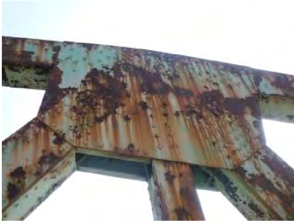
Photo T.21: Span 5, inner west gusset plate at U9. Surface corrosion only. Typical at top chord member gusset plates throughout Span 5.
