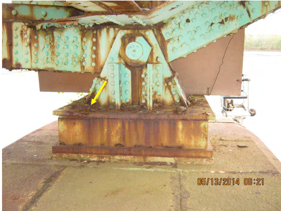
Photo BR.1: Pier 5, fixed bearing under west truss. Typical condition with minor loss in top cover plate and around bearing stiffeners.
