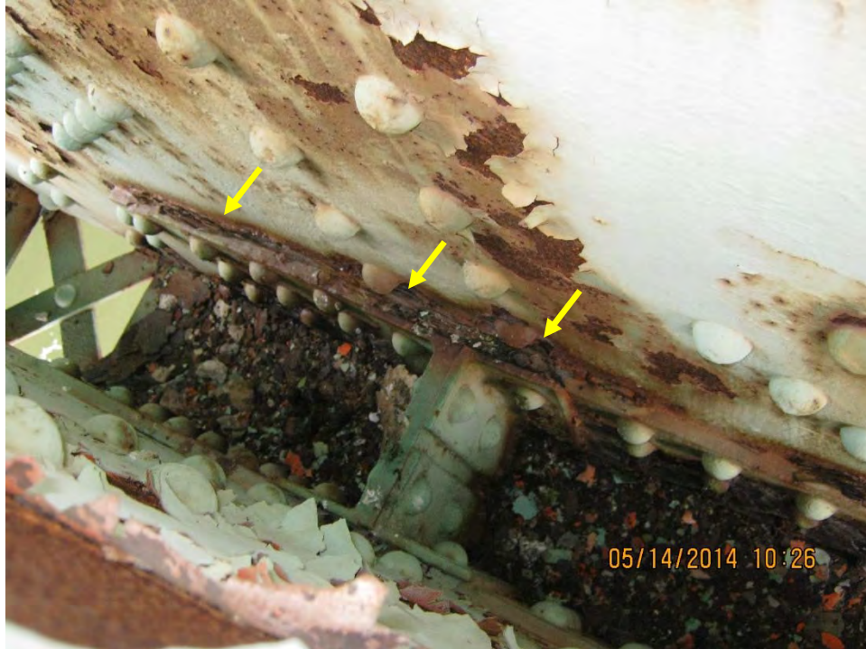
Photo T.19: Span 8, inside of lower gusset plate at L12. Typical loss along the top of diaphragm on the inside of the interior gusset plate.
