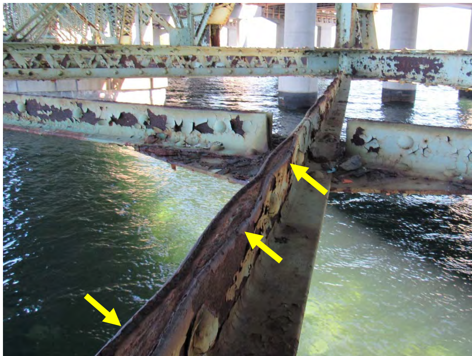
Photo D35: Span 9 Lower Lateral Bracing – Pack Rust Between Double Angles
