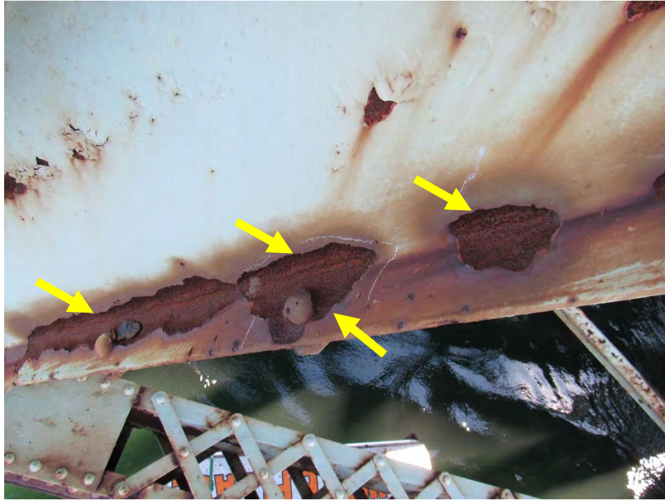
Photo D22: Span 7 – Diagonal Losses at Bottom Flange and Web
