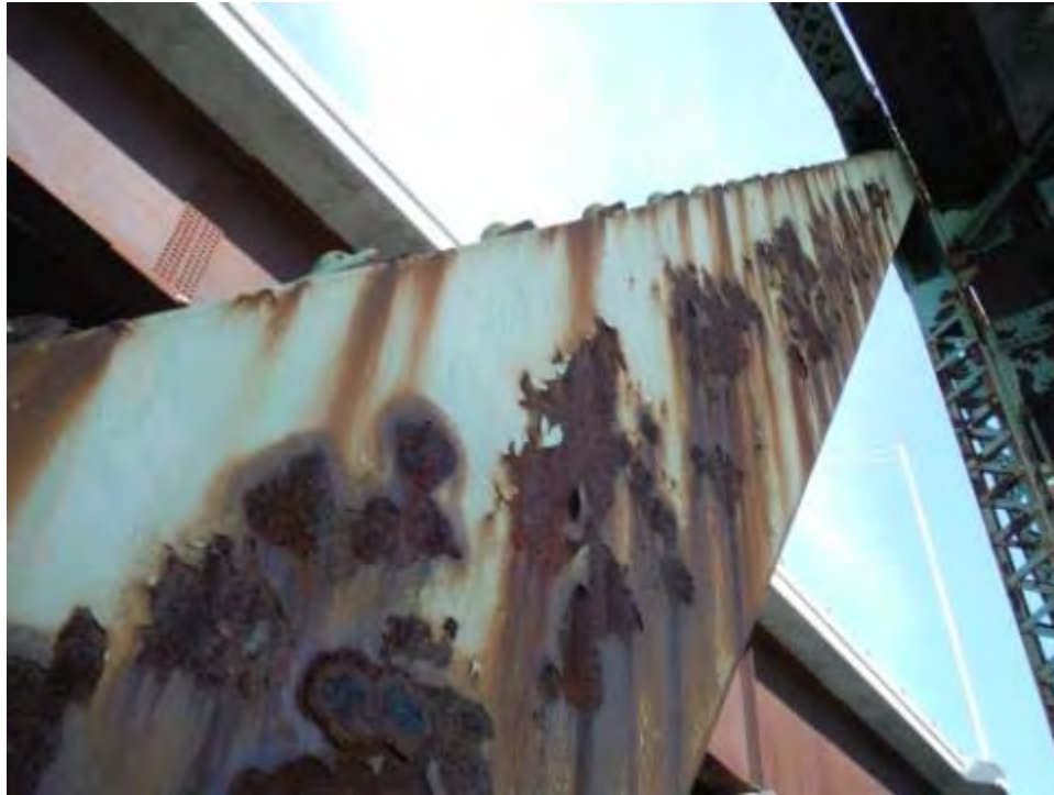
Photo T.9: Span 4, east diagonal L6U7. Random pitting on truss web exterior. Common condition on interior channels throughout the Spans 4, 5 and 6.
