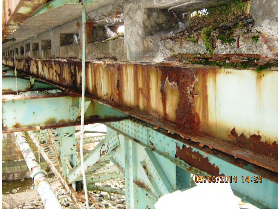
Photo F.1: Span 1, exterior stringers on east fascia directly under deck drains. Typical in poor to serious condition.
