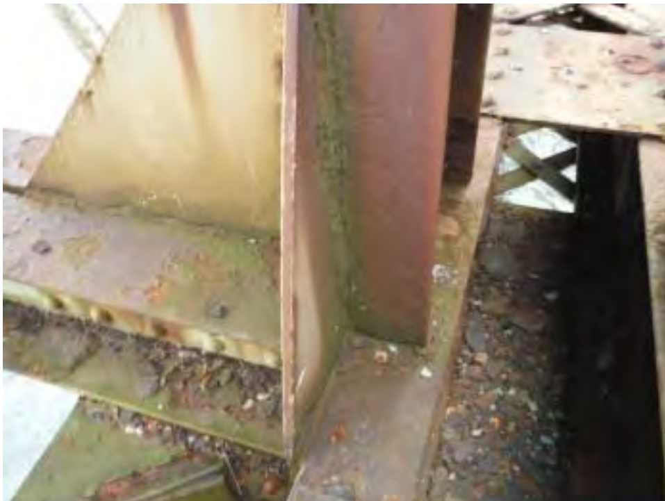
Photo T.6: Span 4, east gusset plate at L3. Section loss and pack rust on gusset plate along interface with bottom chord. Typical condition of diagonal and bottom chord interfaces throughout Spans 4, 5 and 6.
