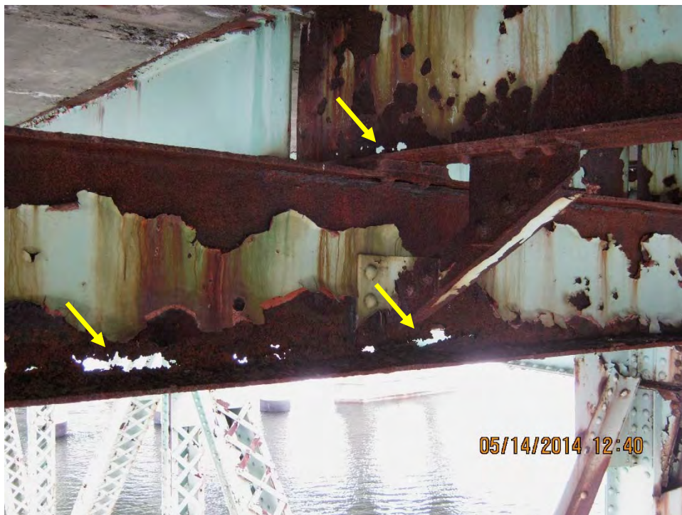
Photo F.8: Span 8, floor beam F14 and interior stringer directly under deck joint. Large areas of full perforation along the bottom of web in floor beam and stringer coupled with flange loss.
