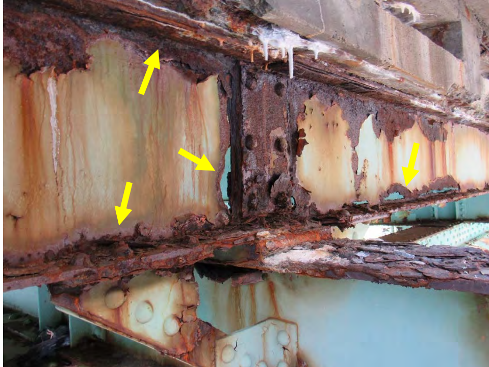
Photo D14: Span 2 Exterior Stringers at Floorbeam Support
