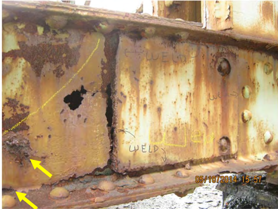
Photo D28: 2014 Inspection – Span 7 East Member L0L1
