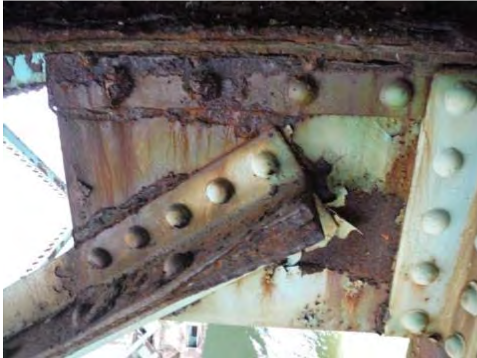
Photo B.7: Span 4, east sway frame gusset plate at U0. Section loss along connection angles to floorbeam bottom flange and truss connections. Typical in many locations throughout the bridge.
