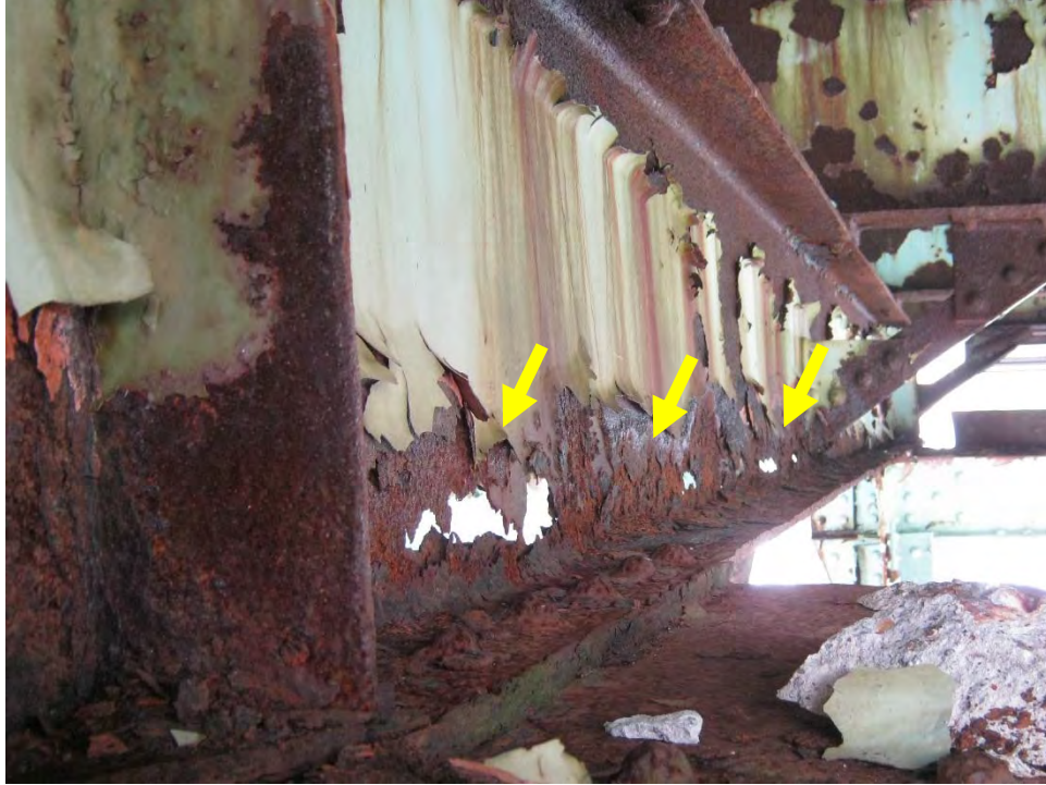
Photo D18: Span 8 – Floorbeam at Deck Joint
