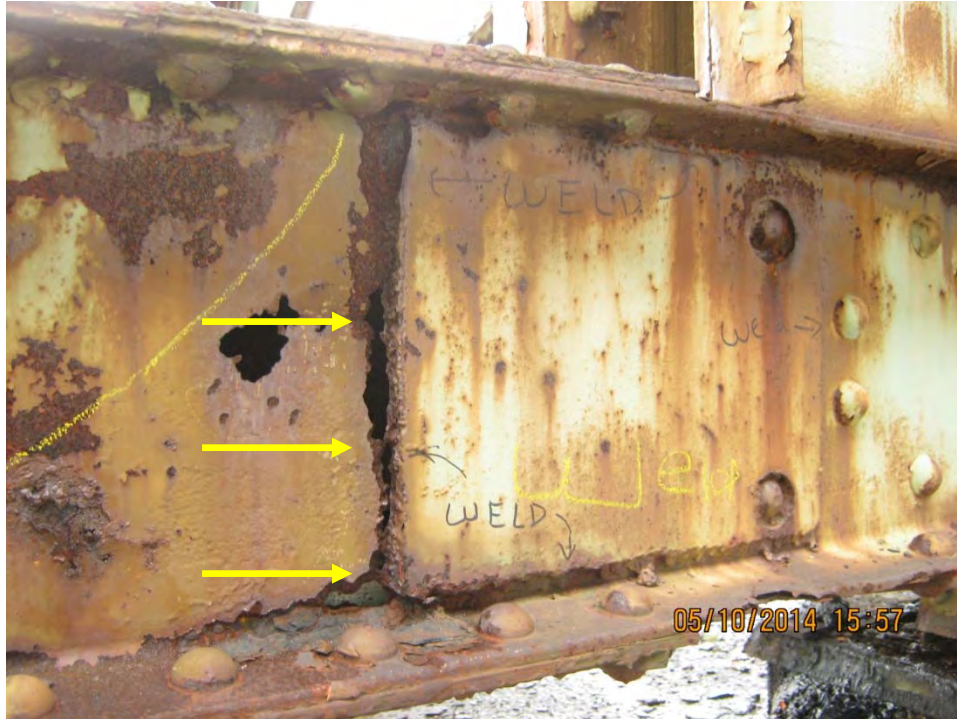
Photo T.14: Span 7, bottom chord member L0L1 of east truss. Full perforation and heavy loss in web along welded retrofit plate in outside channel.
