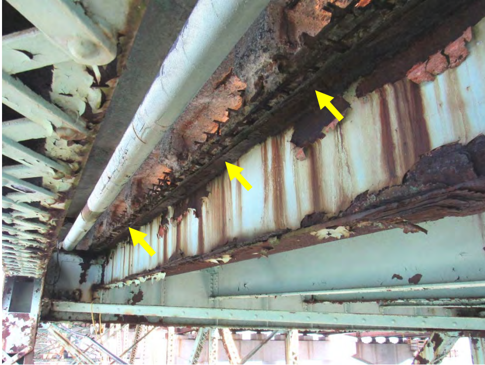
Photo D16: Span 6, West Exterior Stringer Separated From Deck
