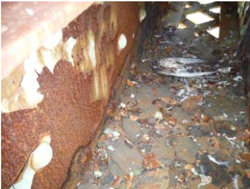
Photo T.8: Span 4, east bottom chord inside L7. Section loss due to laminar corrosion under bottom plate and inside gusset plate connection. Typical condition of bottom chords at gusset plate connections throughout bridge.
