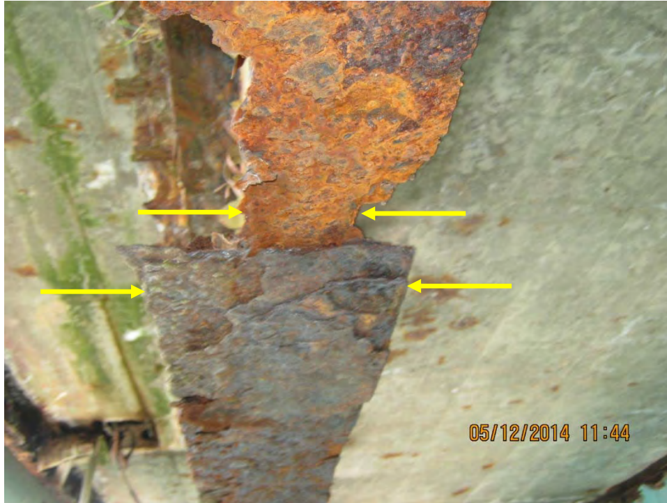
Photo F.3: Span 8, west exterior stringer between F8 and F7. 80% section loss in bottom flange at mid-span.
