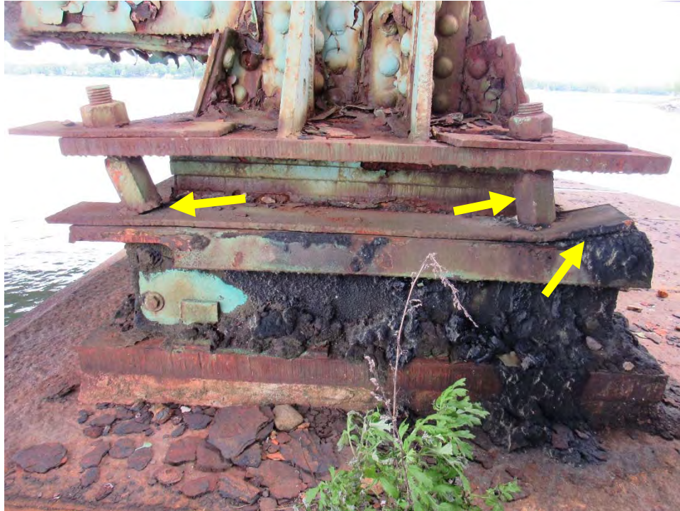
Photo D41: Pier 7 Expansion Bearing – Over-extended With Bent Anchor Bolts
