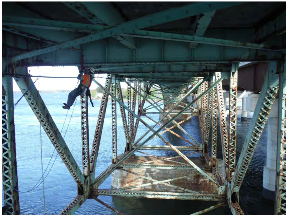
Photo M.2: Industrial rope access was used to inspect the floor system of Spans 3 through 7, and trusses of Spans 4-6.
