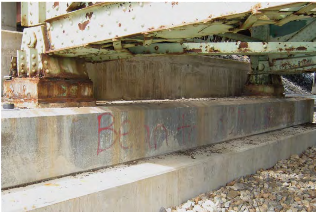
Photo D42: Dover Abutment
