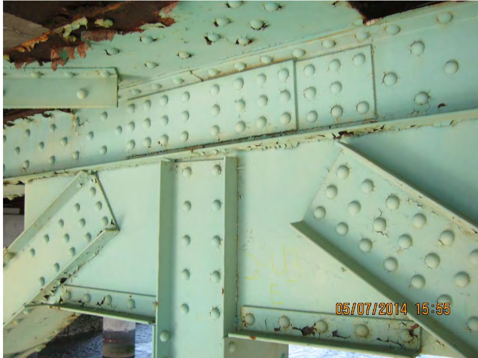
Photo T.20: Span 2, upper gusset plate at U3 on east truss. Upper gusset plates typically in good condition.
