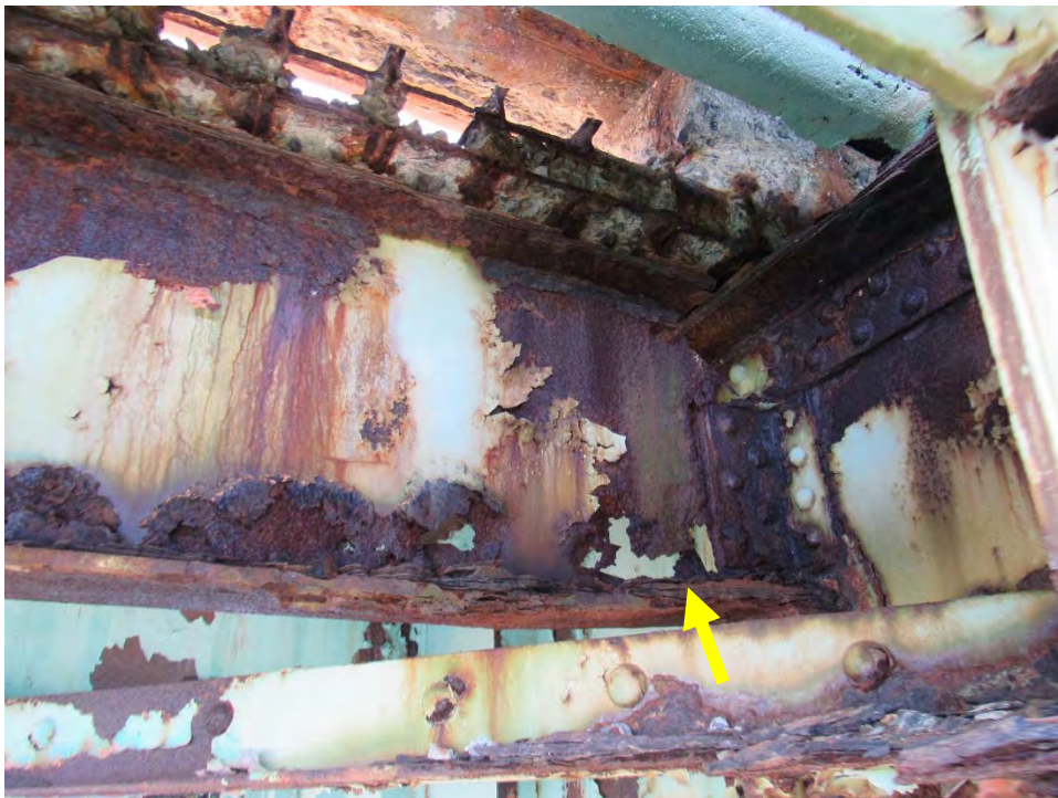
Photo D17: Span 6, West Exterior Stringer – Heavy Section Loss at Floorbeam Connection
