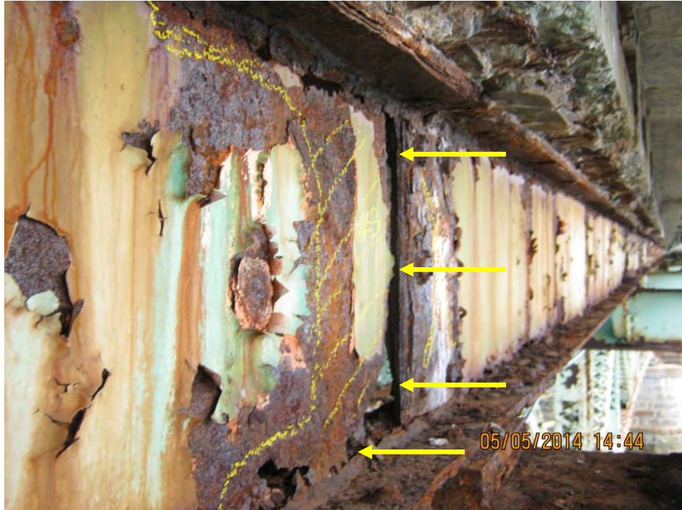
Photo F.4: Span 1, west exterior stringer above F4. Full section loss in the top and bottom of the web and along the connection plate.
