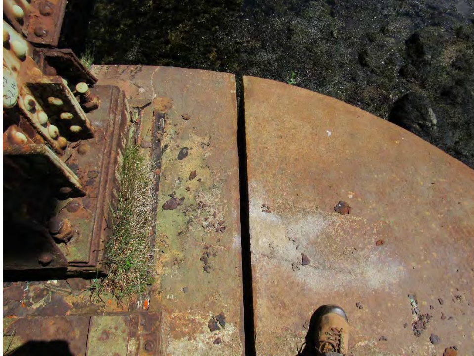
Photo D46: Pier 1 – Missing pointing mortar in cap
