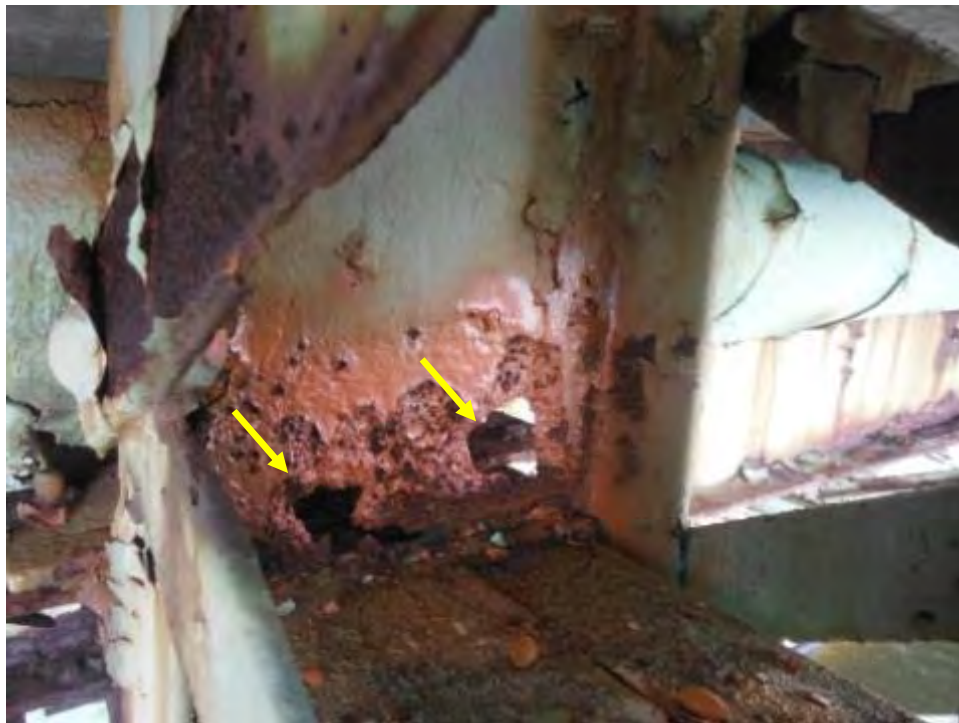
Photo T.4: Span 5, east vertical member U9L9 inner channel web above FB9. Heavy corrosion holes at bottom of hanger. Photo taken of the inside face of U9L9.
