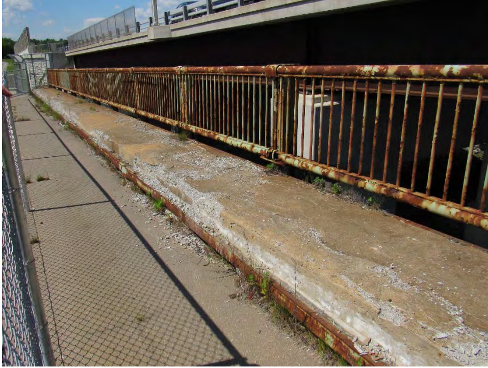
Photo D1: Span 1 and 2 East Sidewalk – Concrete and Railing Deterioration
