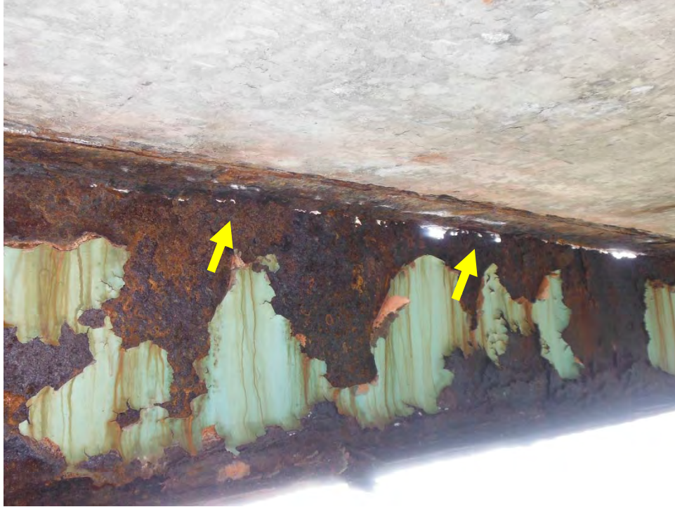
Photo D12: 2014 Inspection - Span 3 Exterior Stringer
