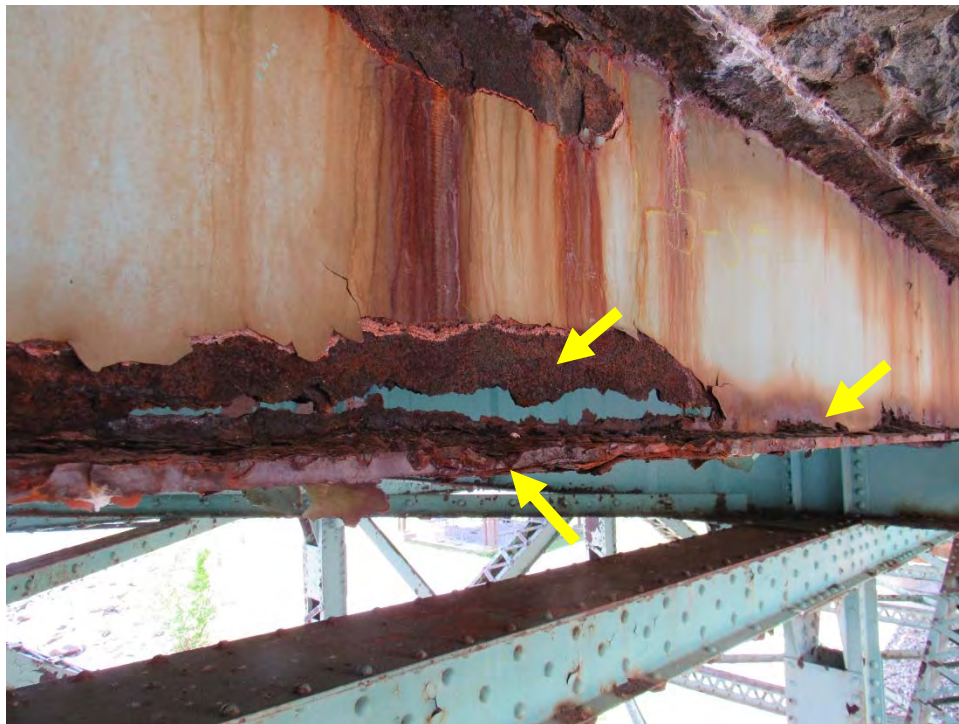
Photo D15: Span 1 Exterior Stringer – Bottom Flange and Web Section Loss
