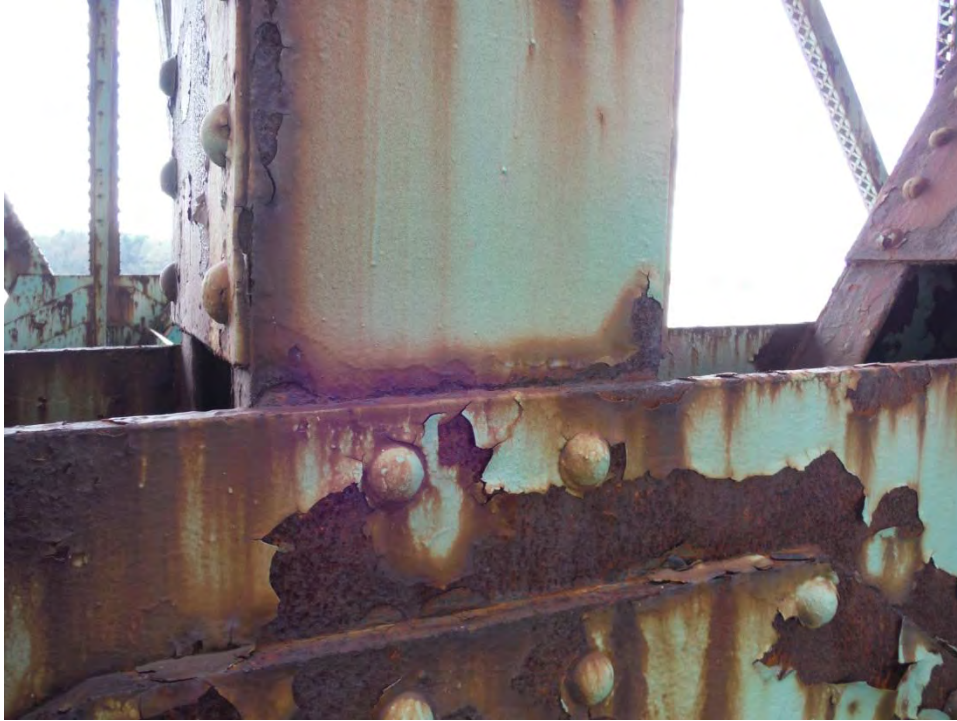
Photo T.5: Span 4, gusset plate at L8 on the east truss. Section loss on vertical L8U8 channel web along gusset plate interface. Typical condition for most lower locations.
