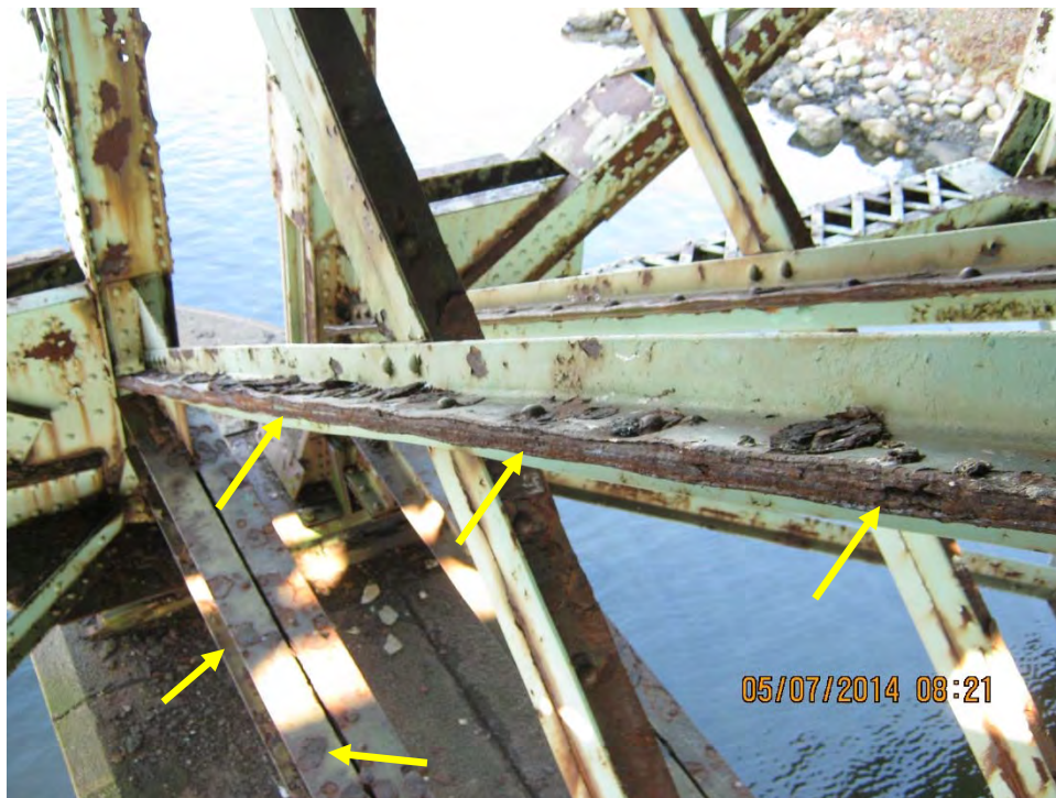
Photo B.3: Pier 1, Span 2, sway bracing below deck joint with heavy pack rust between angles. Pitting on top flanges of lateral strut below.
