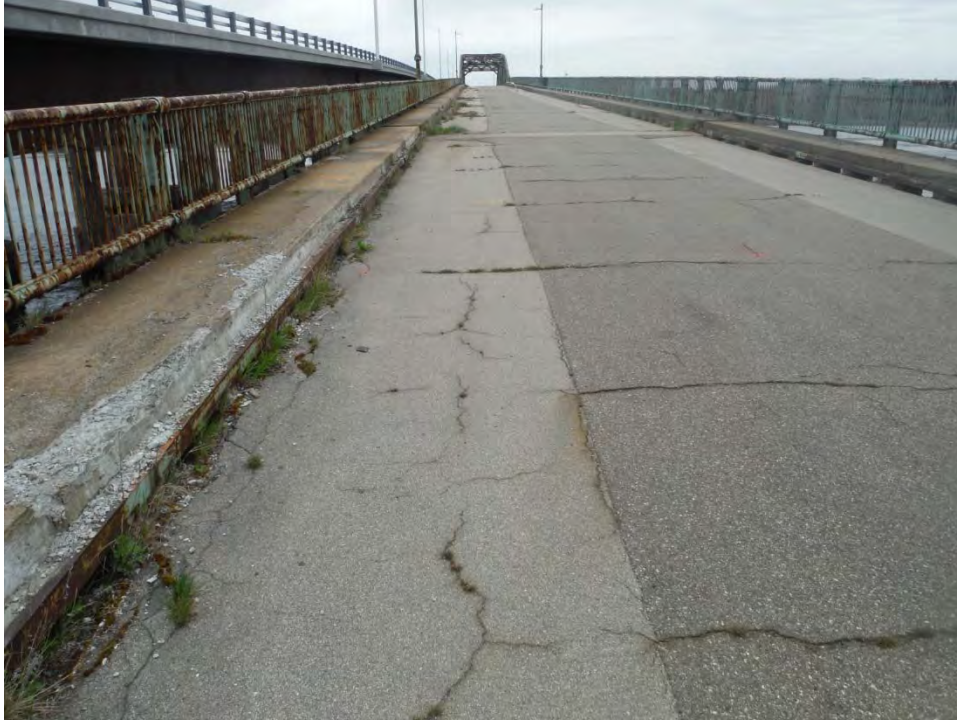
Photo D.3: Bridge looking south from north approach. Cracking in deck wearing surface with vegetation typical throughout bridge.
