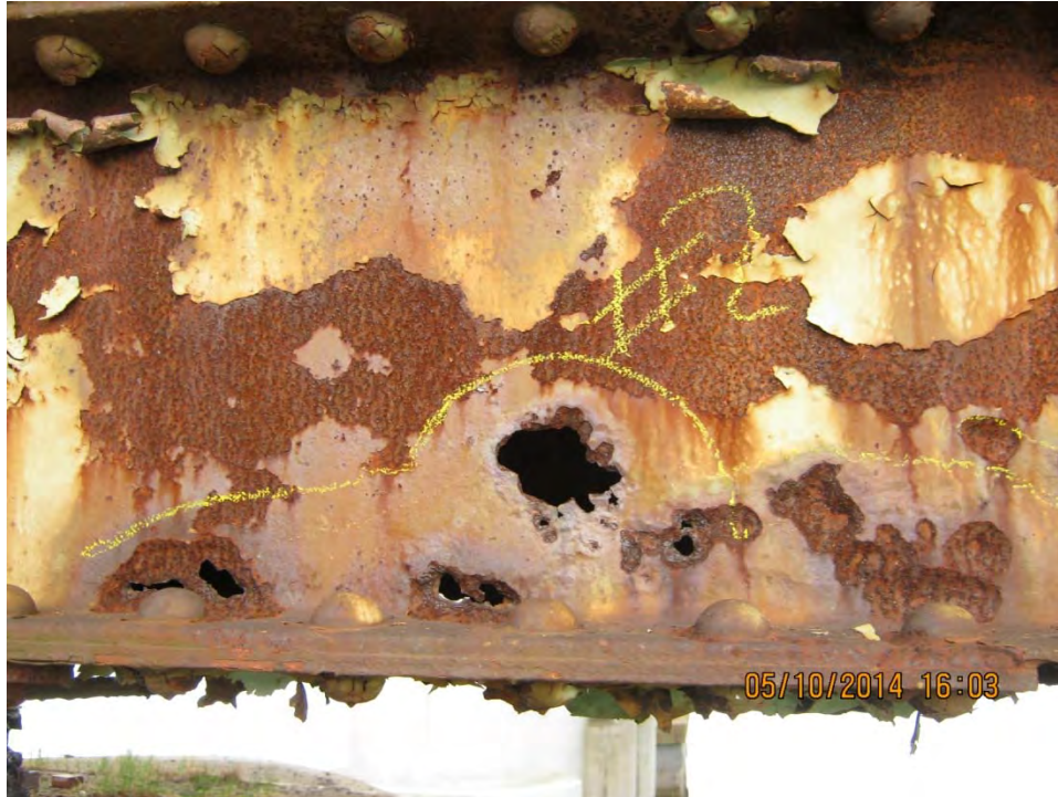
Photo T.15: Span 7, bottom chord member L0L1 of east truss. Several holes surrounded by 50% loss throughout the full height of web in the inner channel.
