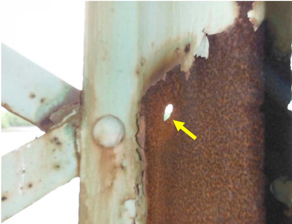
Photo D34: Span 4 Member L3U3 – New Hole in Web
