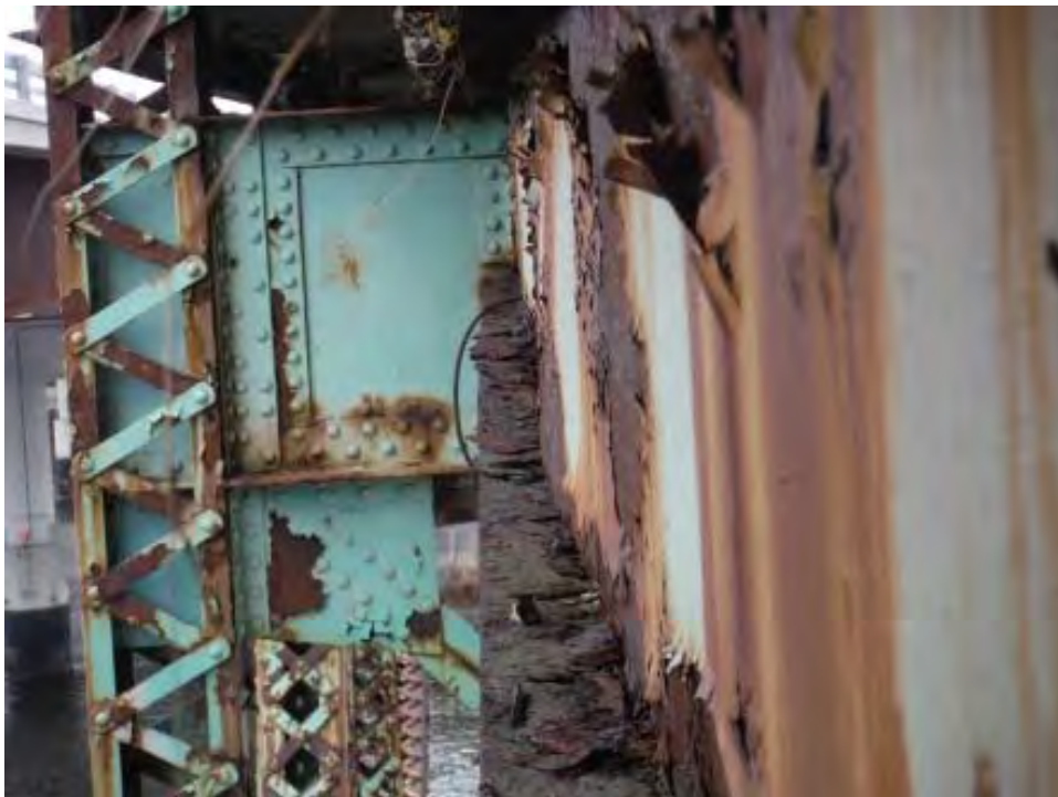
Photo F.6: Span 4, east stringer U7U8. Mid-span buckle on lower web at flange. Due to nearly full-length perforations. Note that a rigging cable had previously been rigged through the hole in the web.
