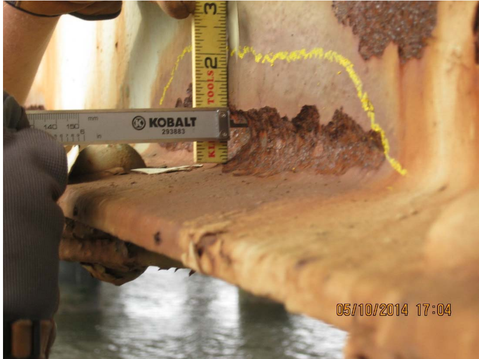
Photo T.2: Span 7, bottom chord member between L7 and L8 on east truss. Typical loss at the bottom of web on channel members.
