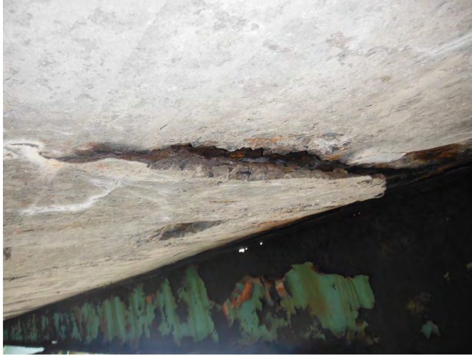
Photo D7: Span 3 – Imminent Deck Spall
