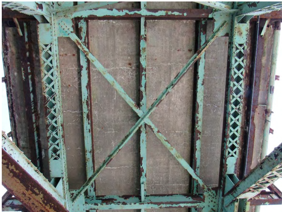
Photo D4: Span 8 – Typical Deck Cracking and Efflorescence
