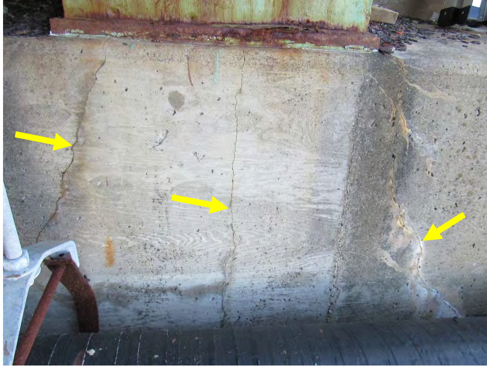
Photo D43: Newington Abutment - Stress Cracks Under West Bearing
