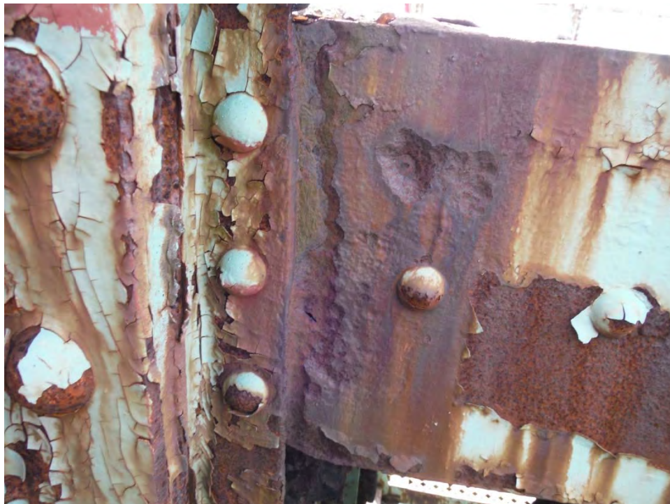
Photo D.10: Span 4, fascia channel at east end of sidewalk deck, located at Floorbeam U1. ¼" pitting full height, along the connection to the bridge railing support. Section loss on fascia channels at railing supports is typical throughout the bridge.
