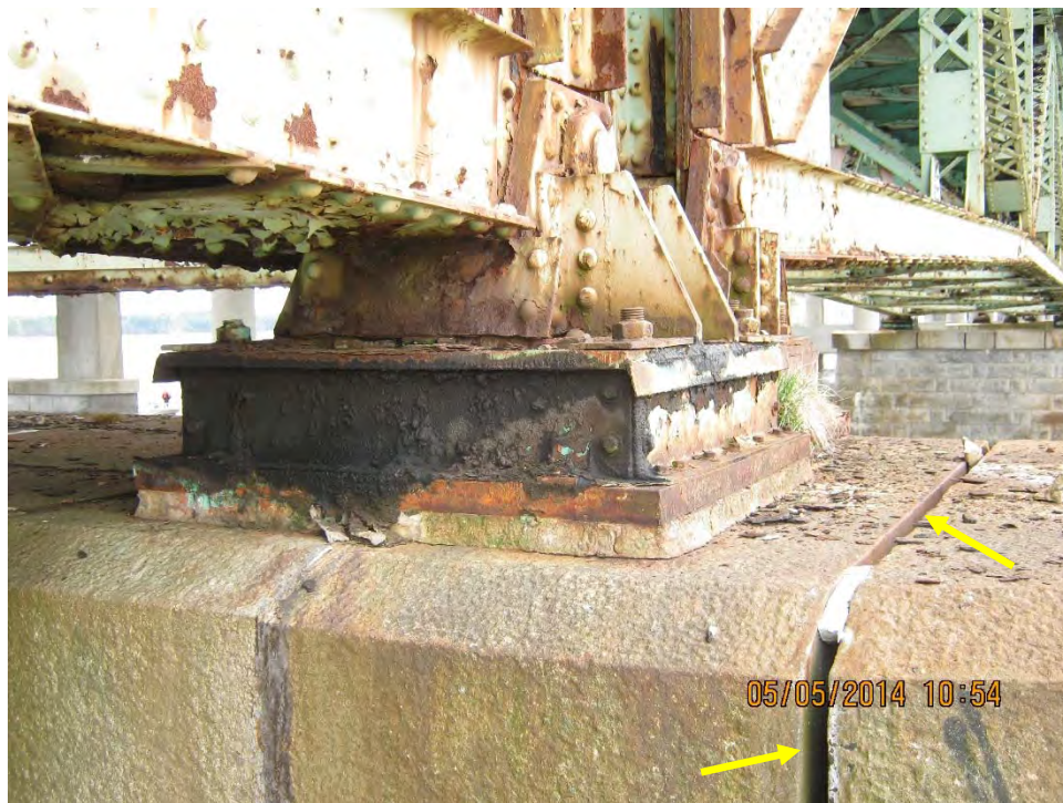
Photo S.3: Pier 1, mortar loss between granite blocks in pier cap. Typical at most piers.
