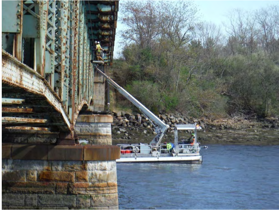
Photo M.1: Proprietary inspection equipment, including the Bucket Boat (shown), and the Tracker (an all-terrain treaded vehicle) were used to inspect Floor systems of Spans 1-2 and 8-9, as well as Trusses of Spans 1-3 and 7-9.
