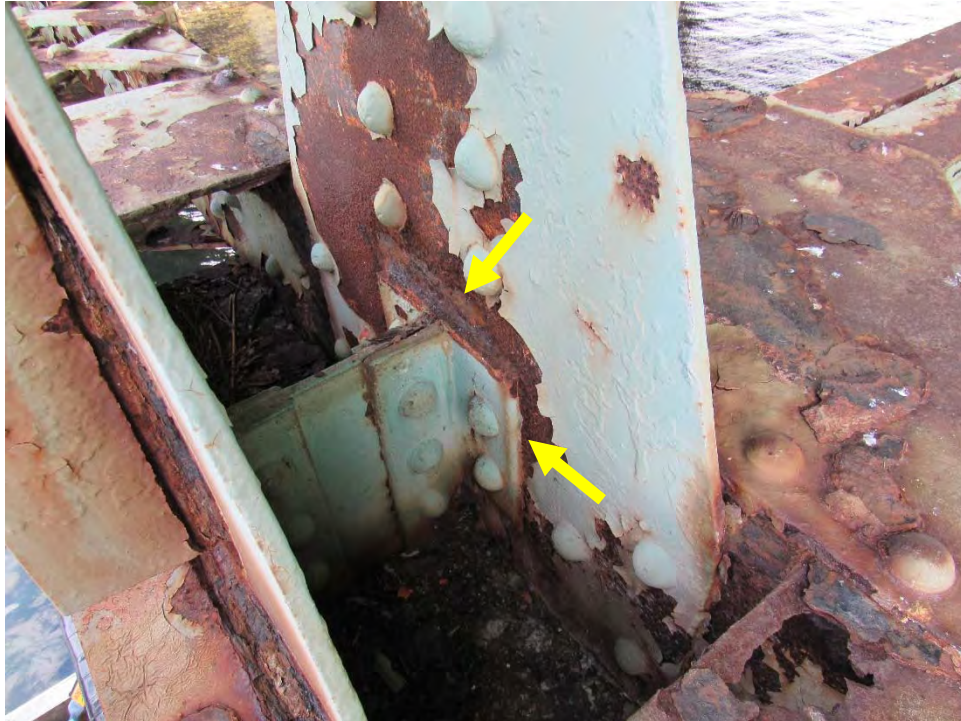
Photo D27: Span 2 Gusset Plate – Section Losses at Interior Stiffener/Diaphragms
