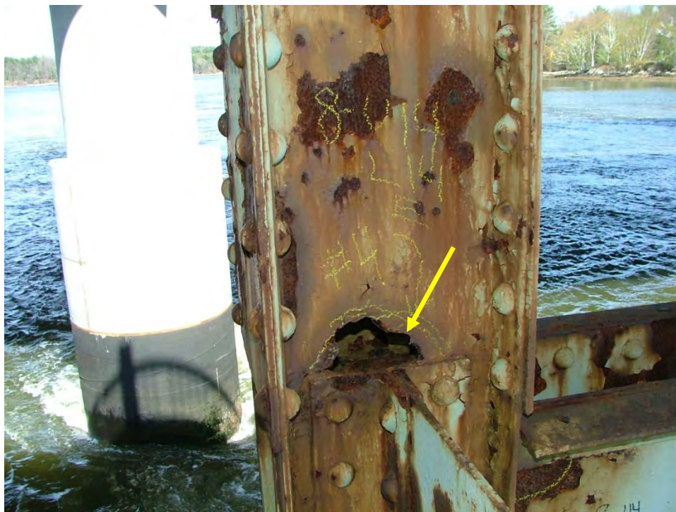
Photo T.16: Span 8, vertical member in east truss at Pier 7. 5" wide hole in web surrounded by 50% loss in full width of web.
