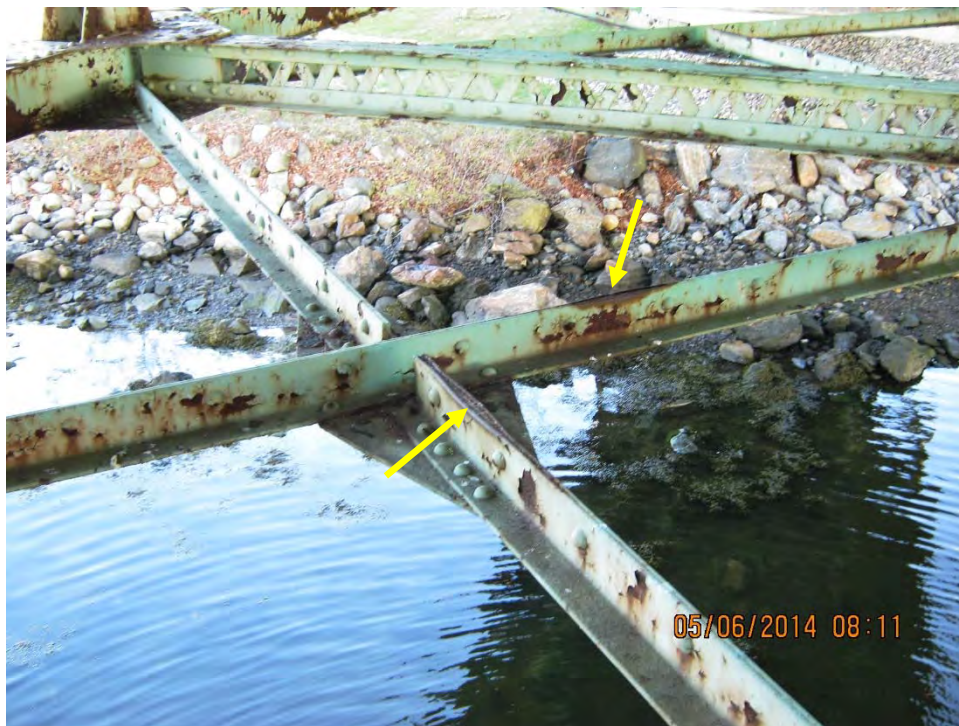
Photo B.1: Span 1, typical bottom lateral bracing condition with pack rust between angles.
