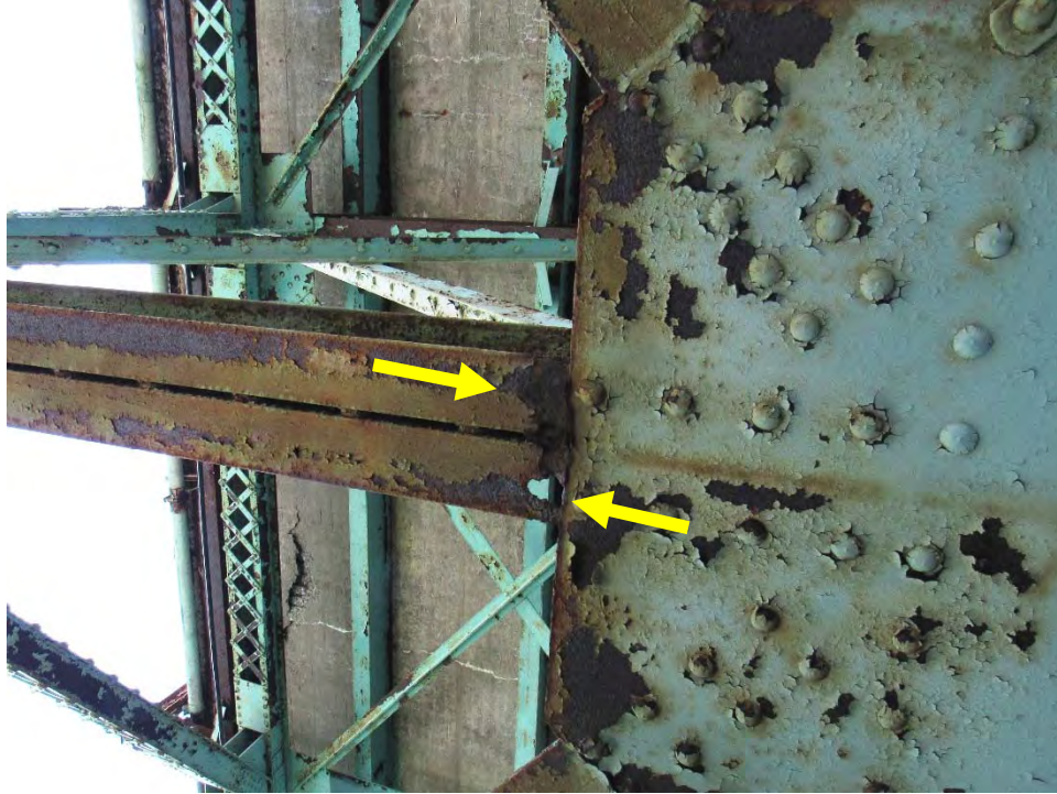
Photo D38: Span 8 Lower Strut of Sway Brace – Section Loss at Connection Plate
