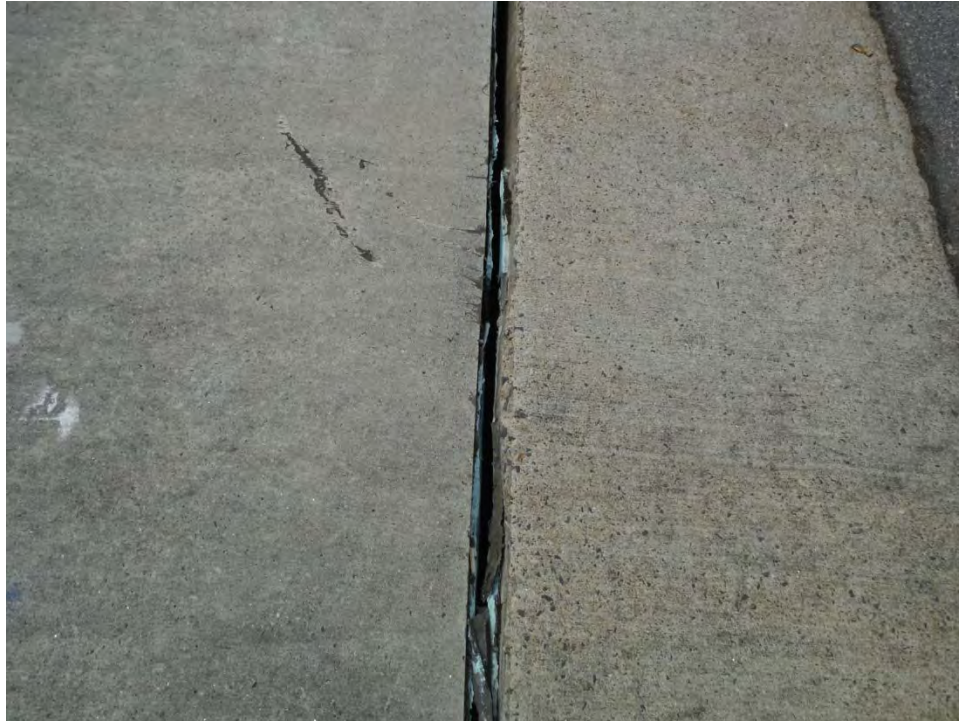
Photo D.7: Deck joint at Pier 6. Joint seal failed full width.
