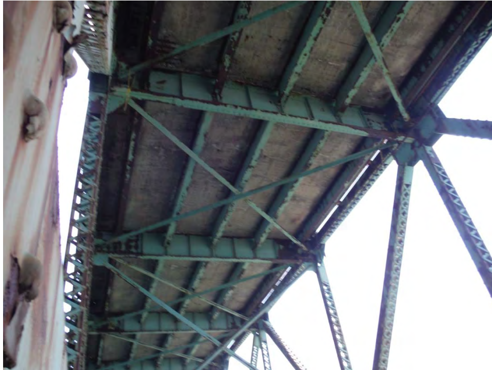
Photo: F.12: Span 6 floor system.
