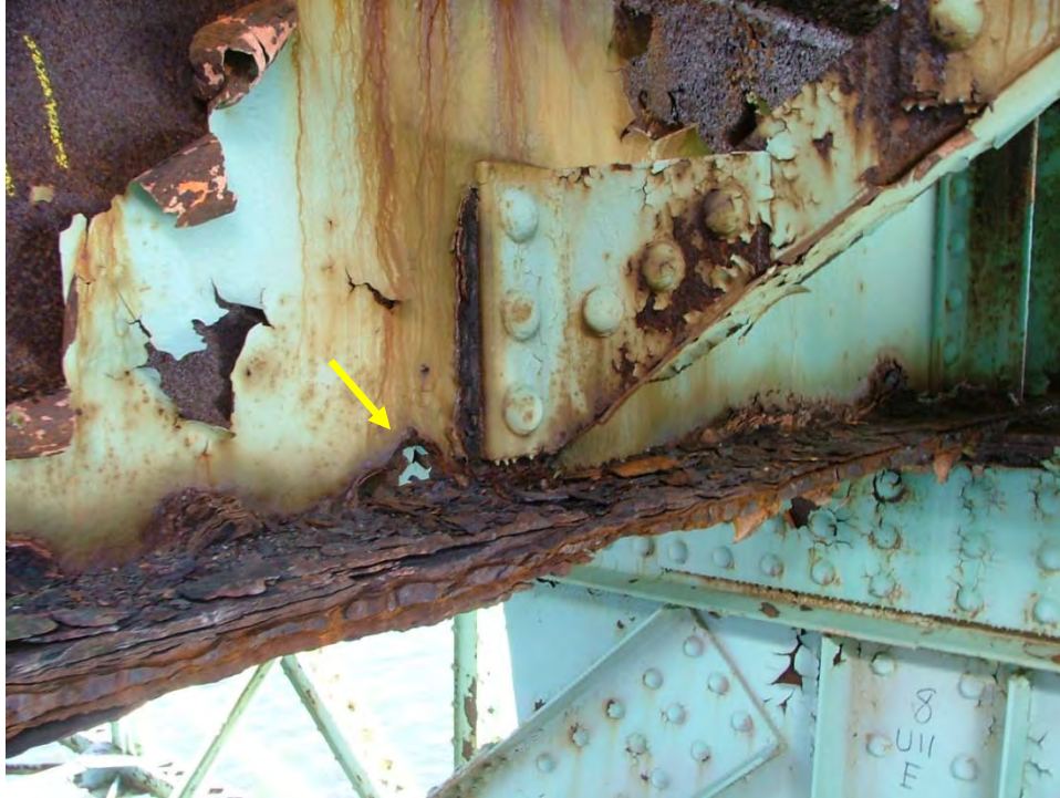
Photo F.7: Span 8, east cantilevered end of floor beam F9. Net thickness of 0.6" in the top and bottom flange with a 2" hole in the web at the exterior stringer knee brace.
