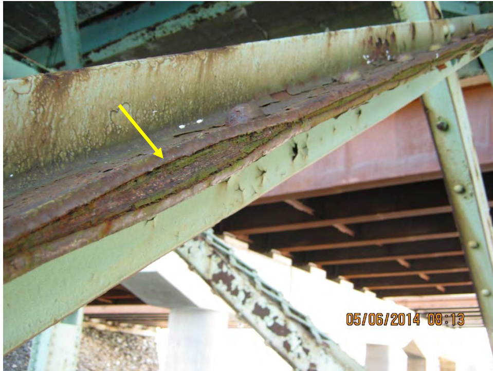
Photo B.6: Pier 1, Span 2, close up view of pack rust between angles, typical on sway and lateral bracing.
