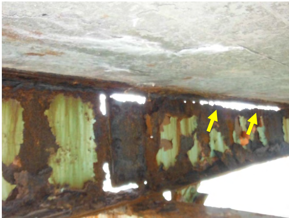
Photo D13: 2016 Inspection – Span 3 Exterior Stringer (Increased Section Loss)
