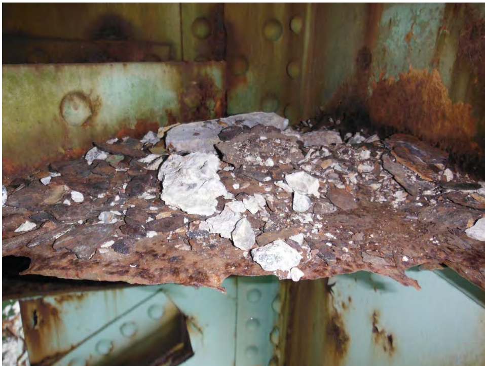
Photo D37: Span 6 – Severe Section Loss in Upper Lateral Bracing Connection Plate
