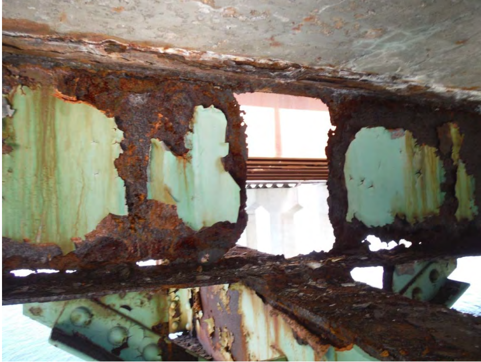
Photo F.5: Span 4, east stringer at FB5. 100% section loss in web at the connection of the two stringers. Connection plate was removed by hand during inspection.
