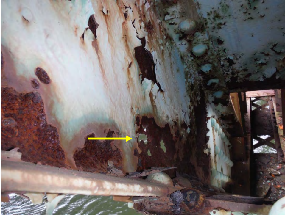
Photo T.13: Span 4, Diagonal L2U1 of the east truss – corrosion holes up to 4½” in diameter on diagonal webs at lower end of chord, adjacent to U1.
