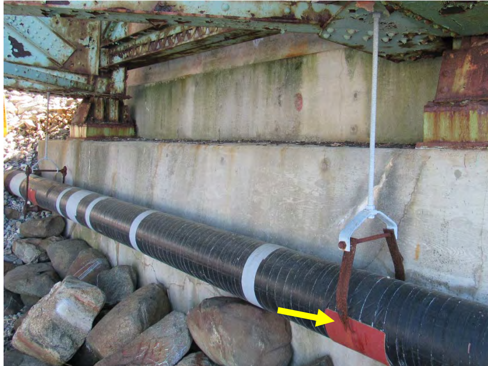
Photo D47: Gas Line – Broken Utility Bracket
