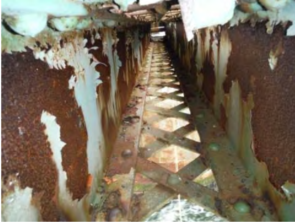
Photo T.7: Span 4, bottom chord L0L1. Surface corrosion and bottom flange section loss inside of chord. Typical throughout all truss members.
