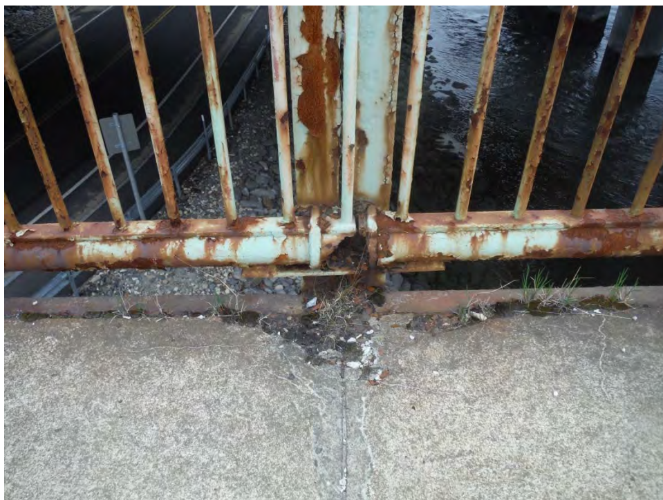
Photo D.8: Span 1, bridge railing and post. Up to 100% section loss in lower rail, and over 50% section loss in post flanges typical throughout bridge.
