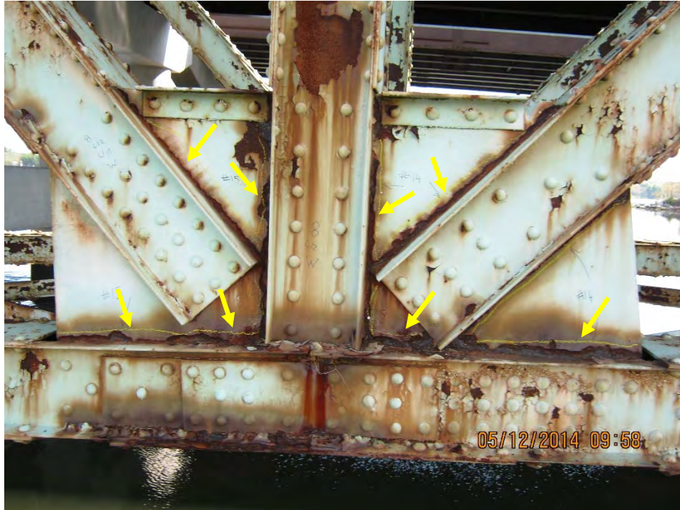
Photo T.18: Span 8, lower gusset plate at L12 on west truss. Typical losses along the bottom chord, diagonal, and vertical members.
