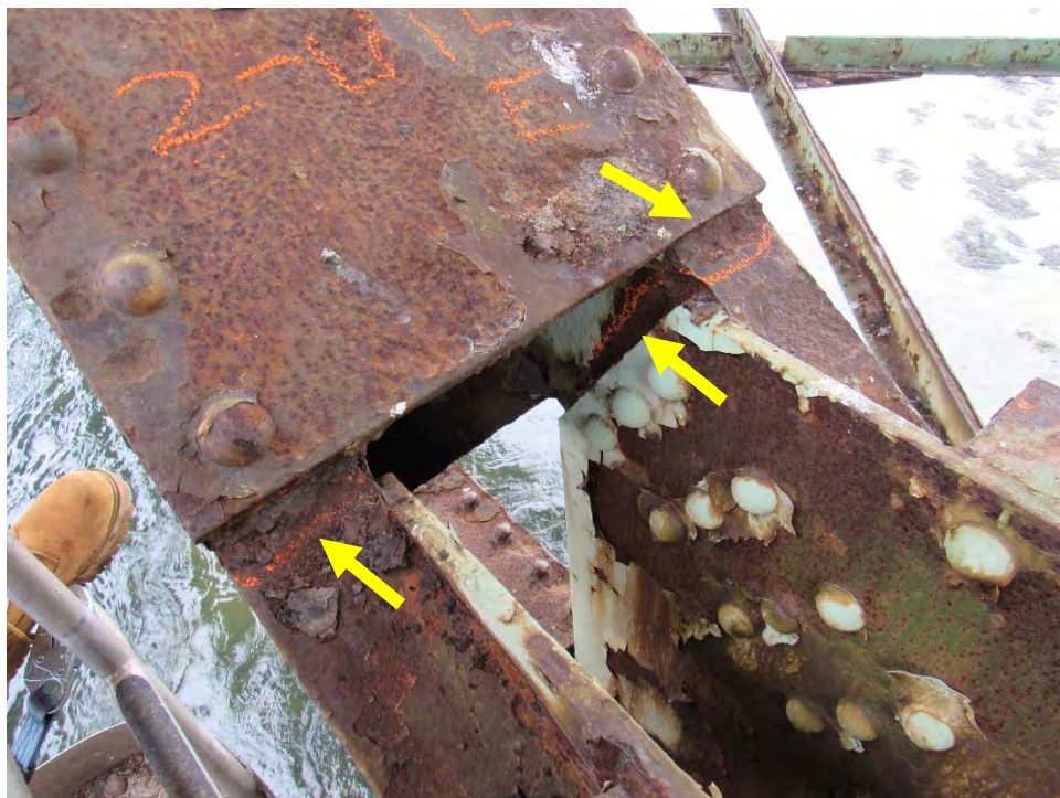
Photo D23: Span 2 Diagonal Member - Losses at Gusset and Batten Plate Connections
