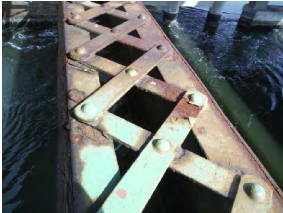
Photo T.12: Span 5, east bottom chord L12L13. Pack rust and section loss to lacing bars. Typical throughout the bridge.
