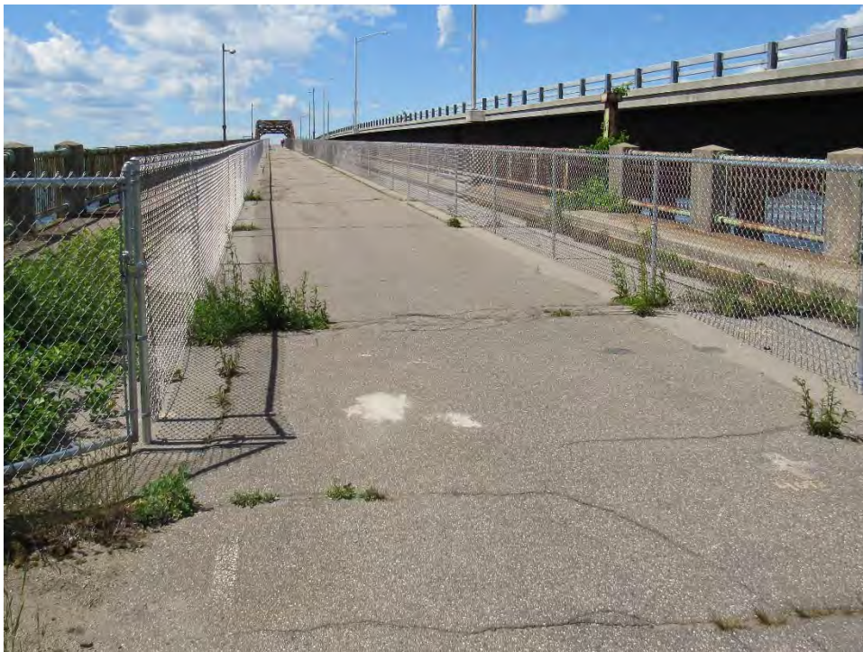
Photo D2: Top of Deck at Newington Abutment Looking North
