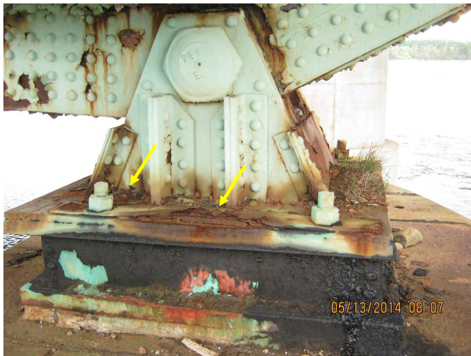
Photo BR.2: Pier 4, expansion bearing under west truss. Typical condition with minor loss in top cover plate and around bearing stiffeners.
