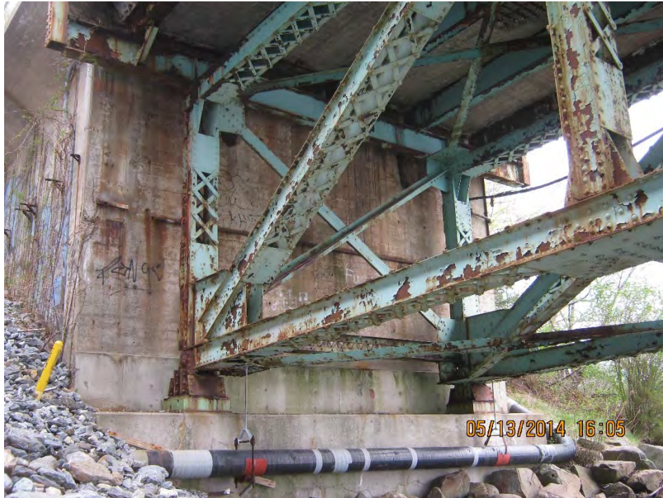
Photo S.2: Newington abutment and wingwalls in overall good condition.
