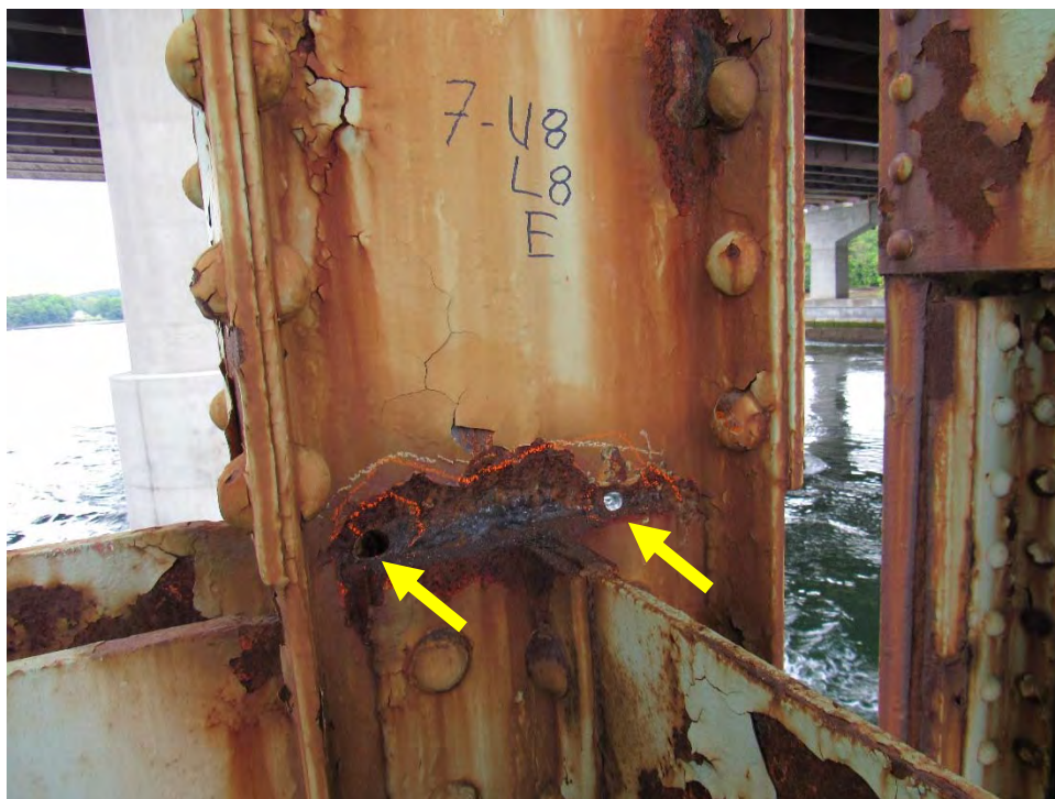
Photo D33: 2016 Inspection – Span 7 East Member L8U8 (New Holes)
