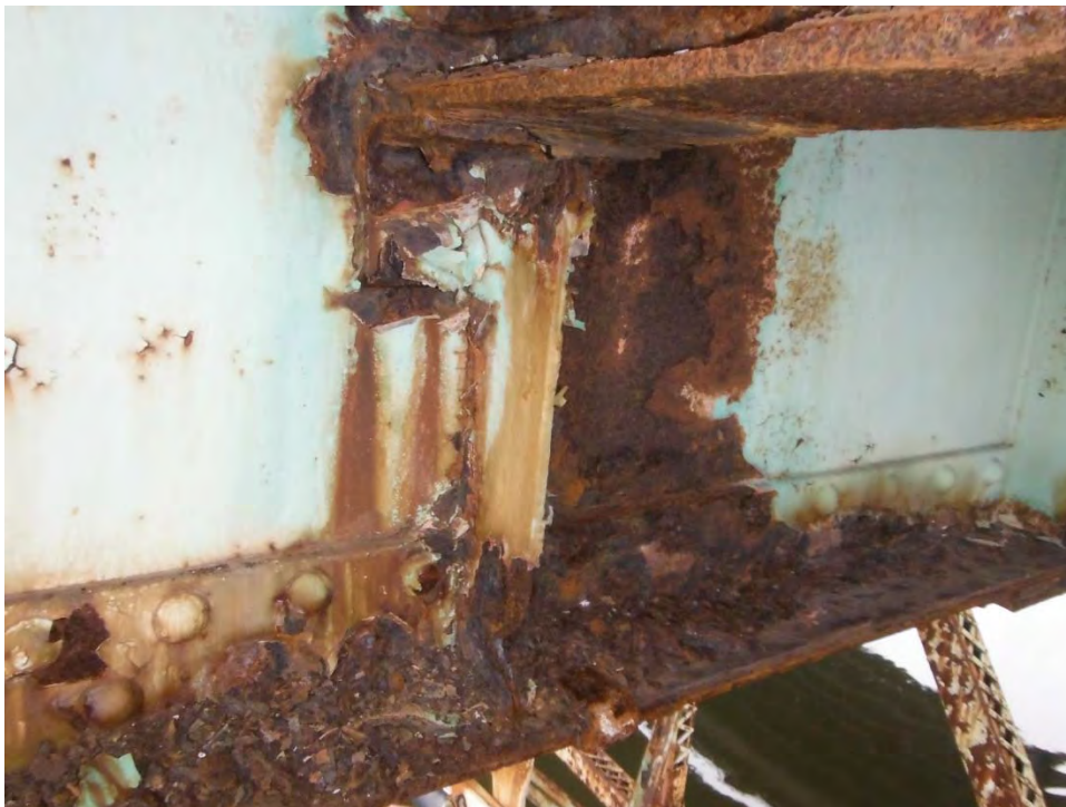
Photo F.10: Span 6, Floorbeam 8 at west stringer. Section loss in floorbeam at ends with holes in stiffeners typical.
