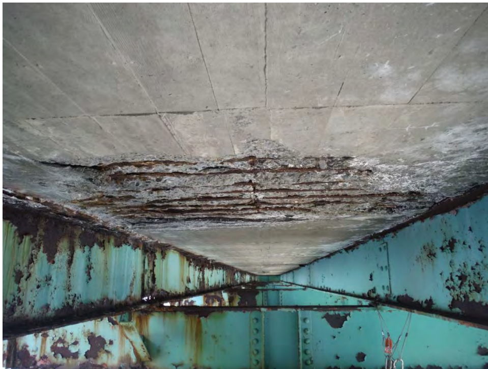
Photo D.2: Span 3, deck at mid-panel between Floorbeams 8 and 9, also between Stringers 4 and 5. Typical spalling in deck, exposed rebar with section loss.
