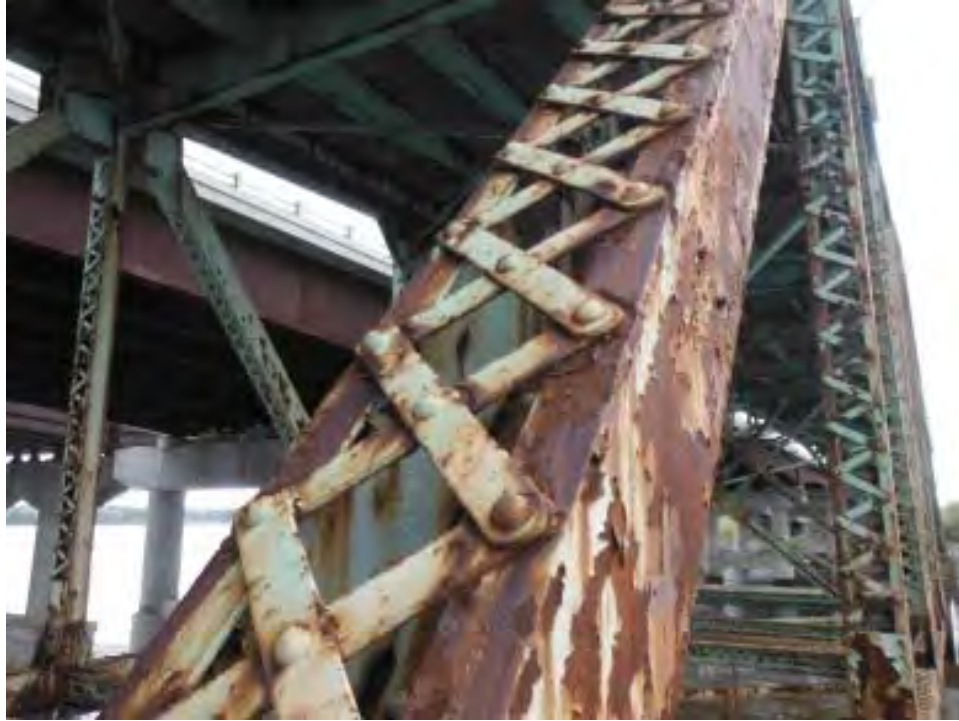
Photo T.11: Span 4, west diagonal truss member U5L4. Section loss on flange at lacing bars. Section loss at interface with lacing bars typical for most channel flanges on top and bottom throughout the bridge.
