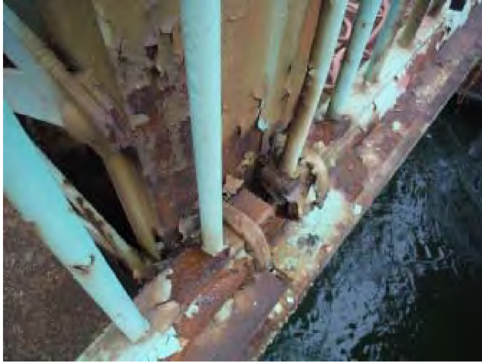
Photo D.9: Span 5, railing at top of east vertical member L11'-U11'. Section loss to exterior web of vertical channel. Similar condition throughout Span 5
