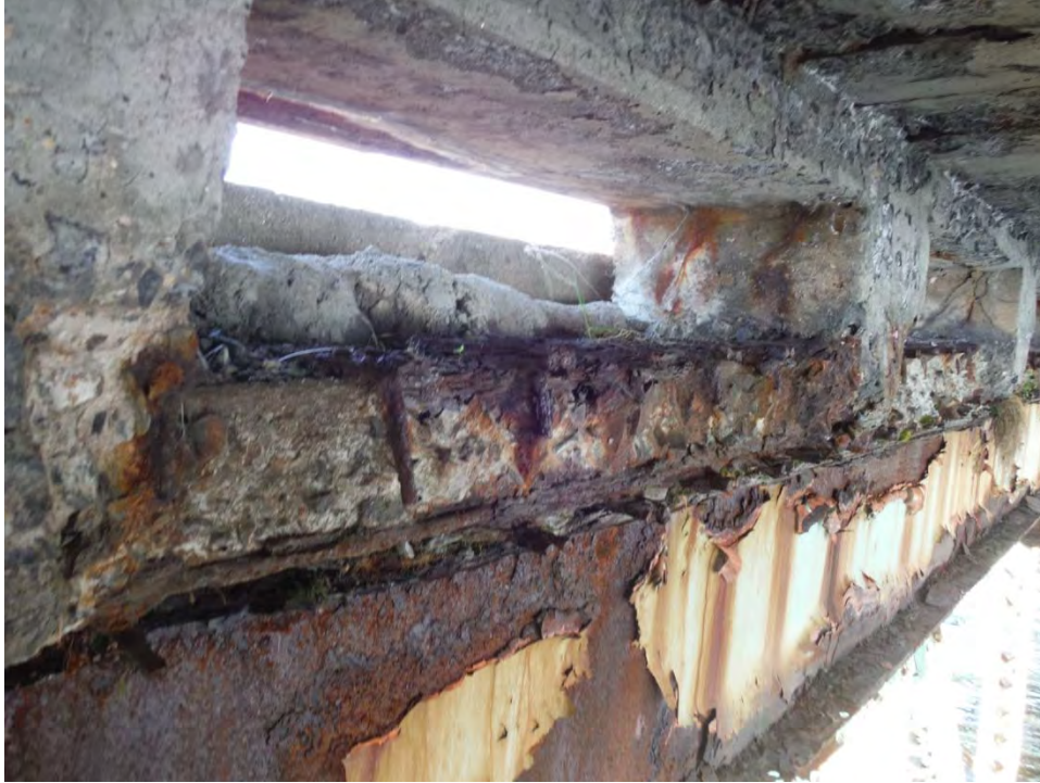
Photo D.1: Span 7, East end of deck at deck drains. Severe spalling and up to 100% section loss in rebar at ends typical.
