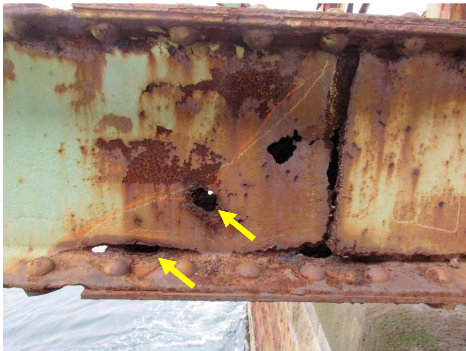
Photo D29: 2016 Inspection – Span 7 East Member L0L1 (New Holes and Section Loss)
