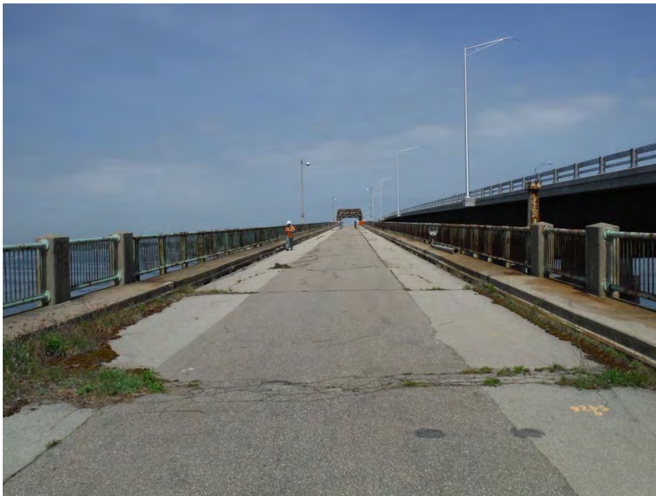
Photo D.4: Bridge looking north from south approach.
