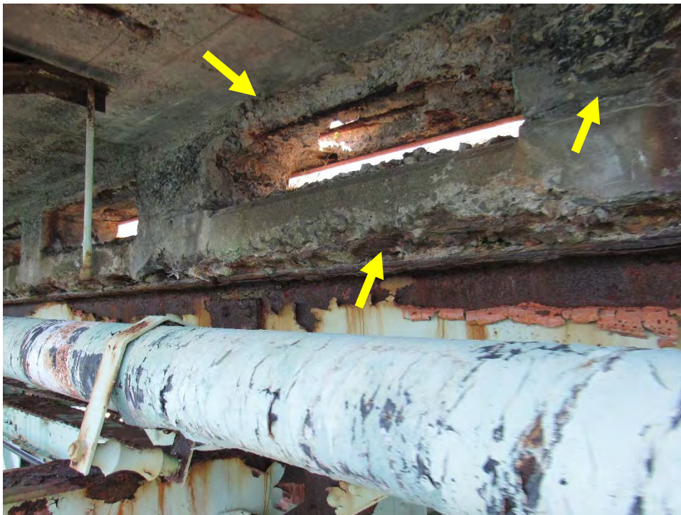
Photo D6: Span 6 – Spalls and Exposed Rebar at Curb Openings
