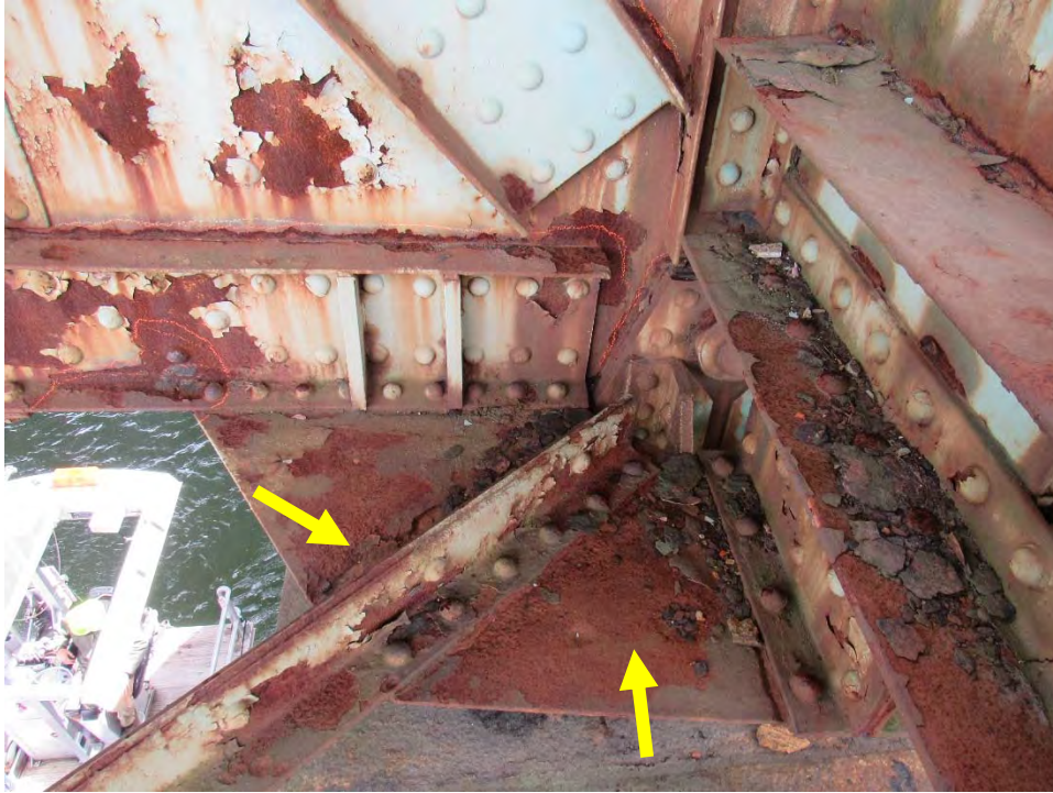
Photo D36: Span 3 Lower Lateral Bracing and Connection Plate Deterioration
