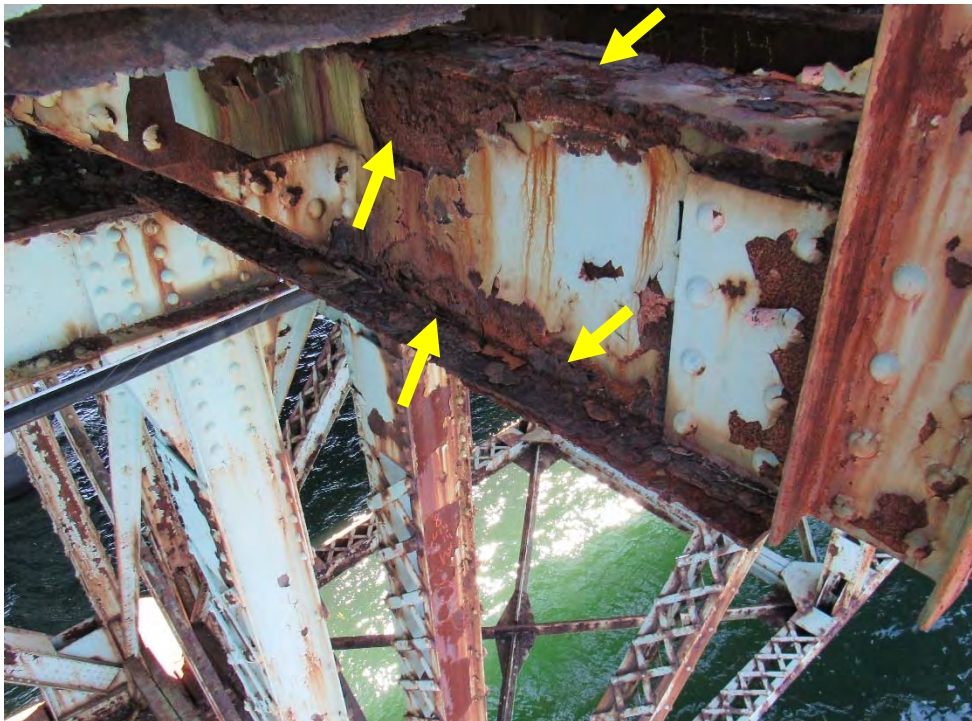
Photo D19: Span 8 Floorbeam – Section Loss at End Region
