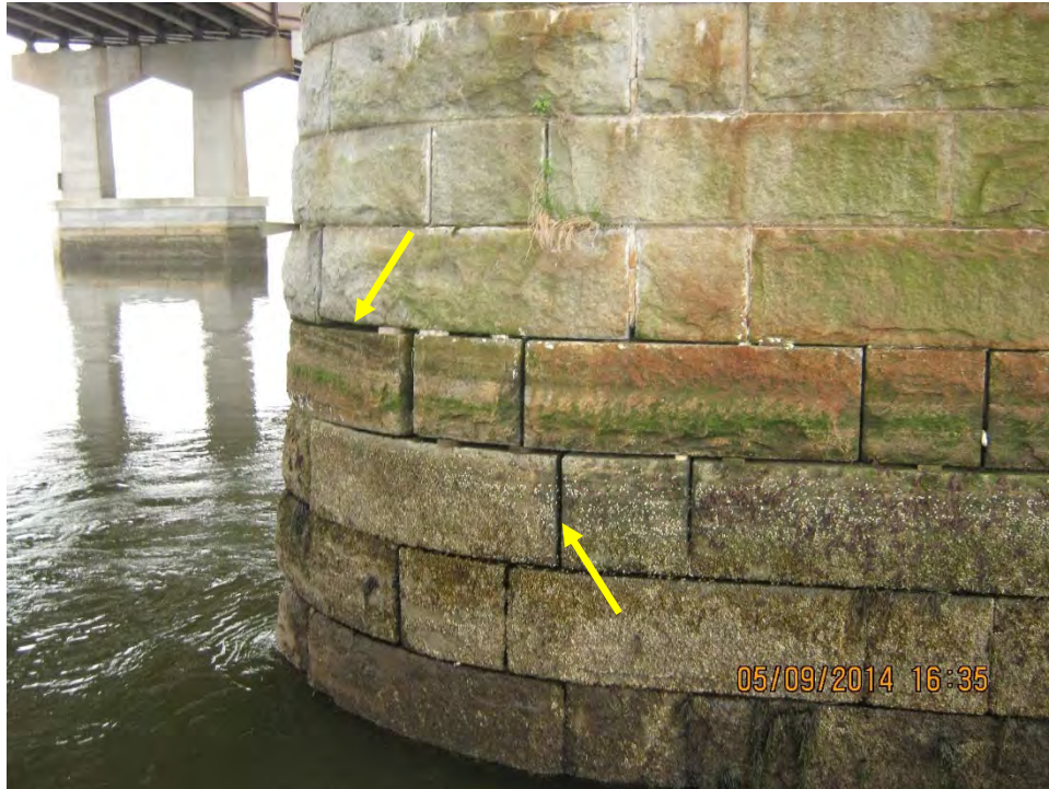
Photo S.4: Pier 3, heavy mortar loss between granite blocks below water level. Typical condition for most piers.
