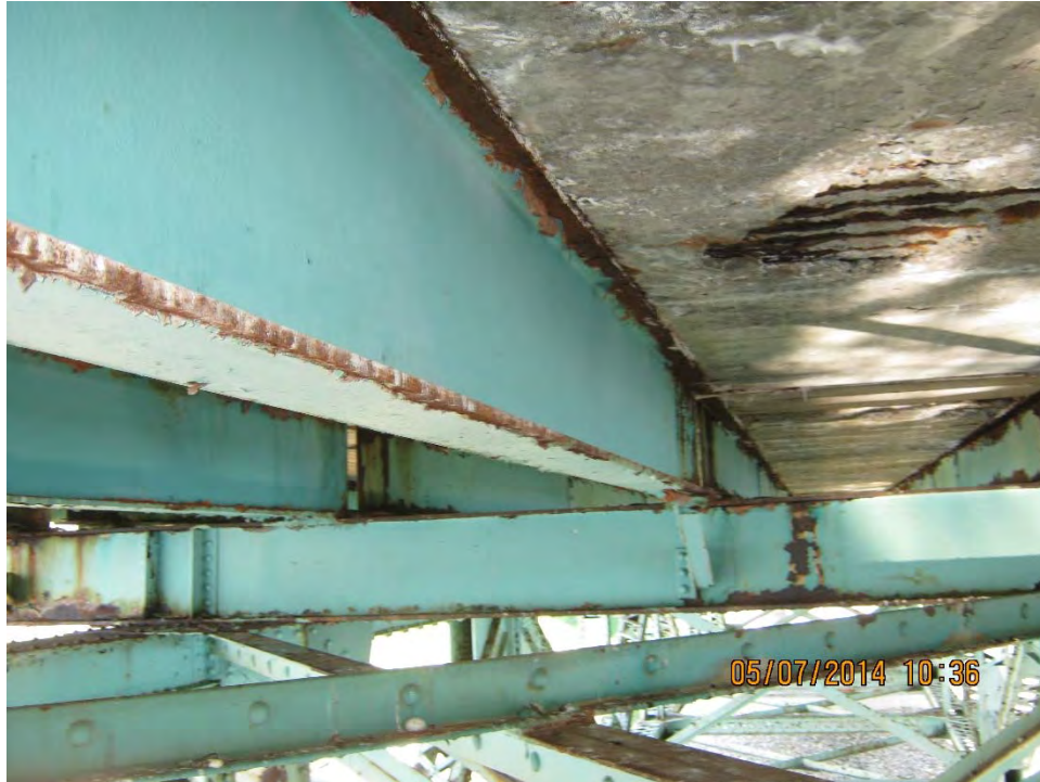
Photo F.2: Span 2, interior stringers and interior of floor beams typically in fair condition.
