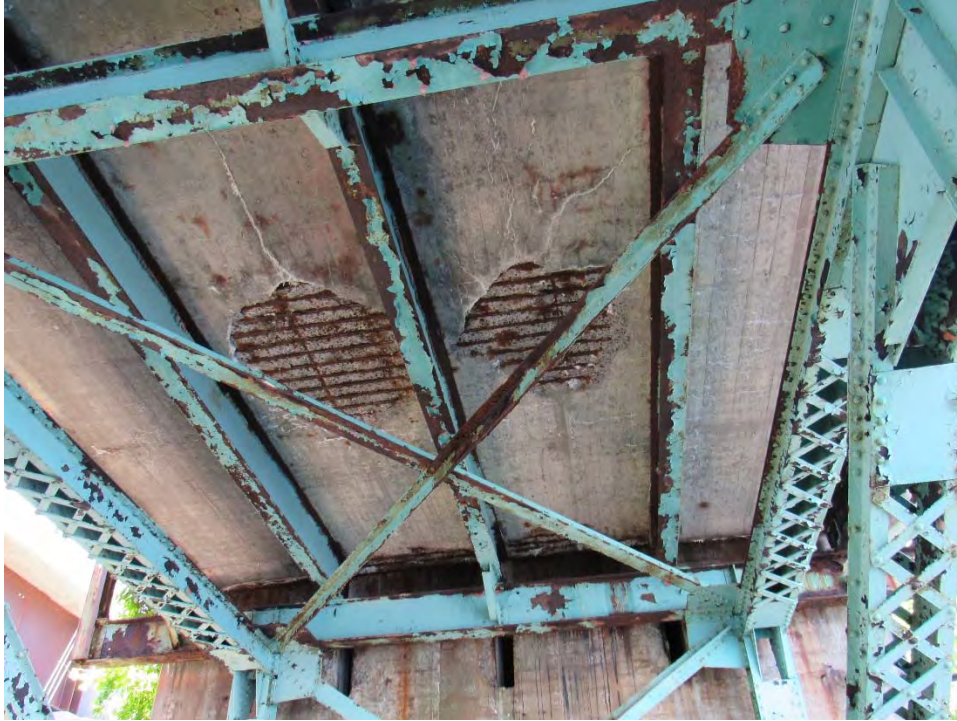
Photo D5: Span 9 - Spalled Deck Areas with Exposed Rebar
