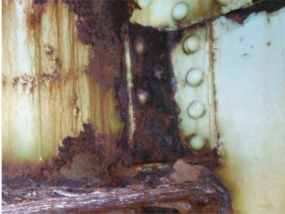
Photo D10: 2014 Inspection - Span 6 Exterior Stringer
