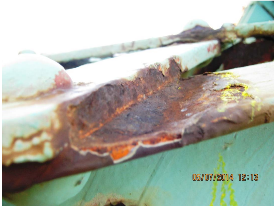
Photo T.1: Span 2, diagonal member between L6 and U5 on east truss. Typical loss on top flange of channel member at lacing bar.
