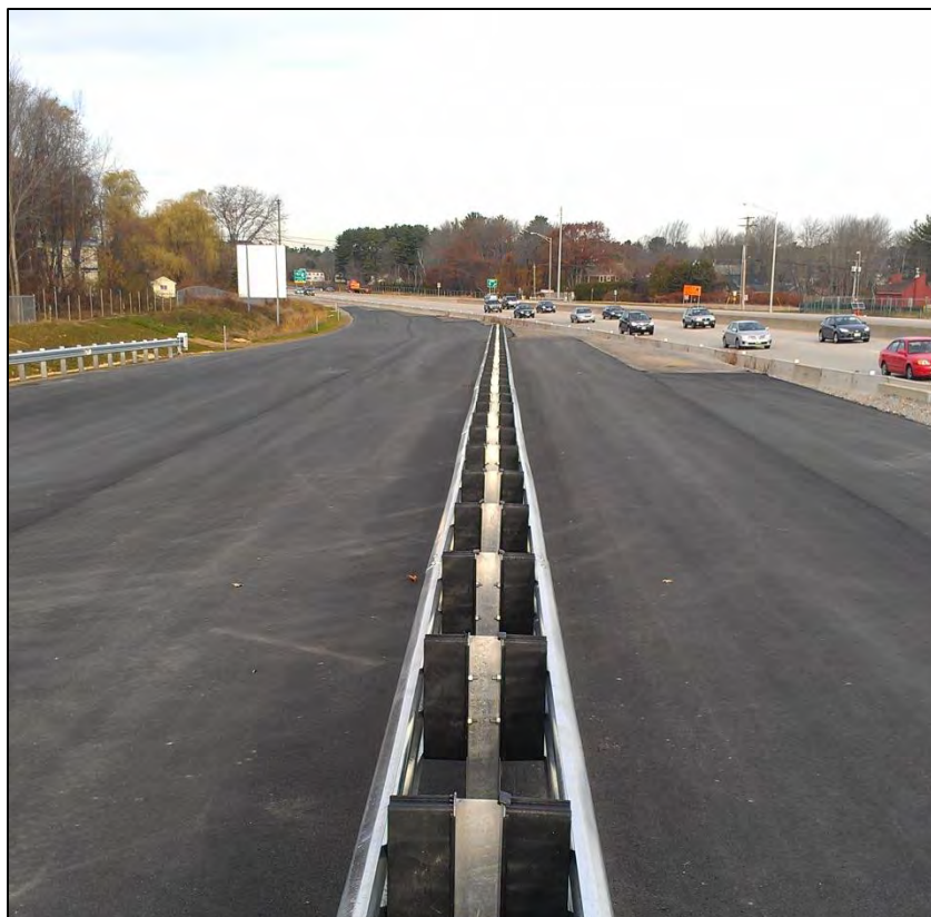
Photo Date: 09/30/14- Approach to the New Little Bay Bridge.
