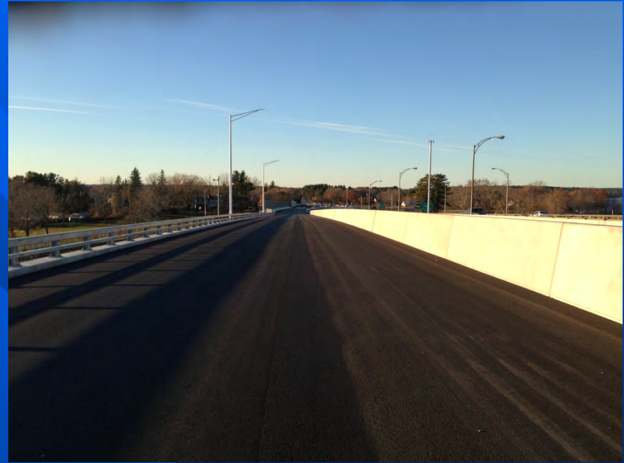
Final Bridge Deck (2013)
