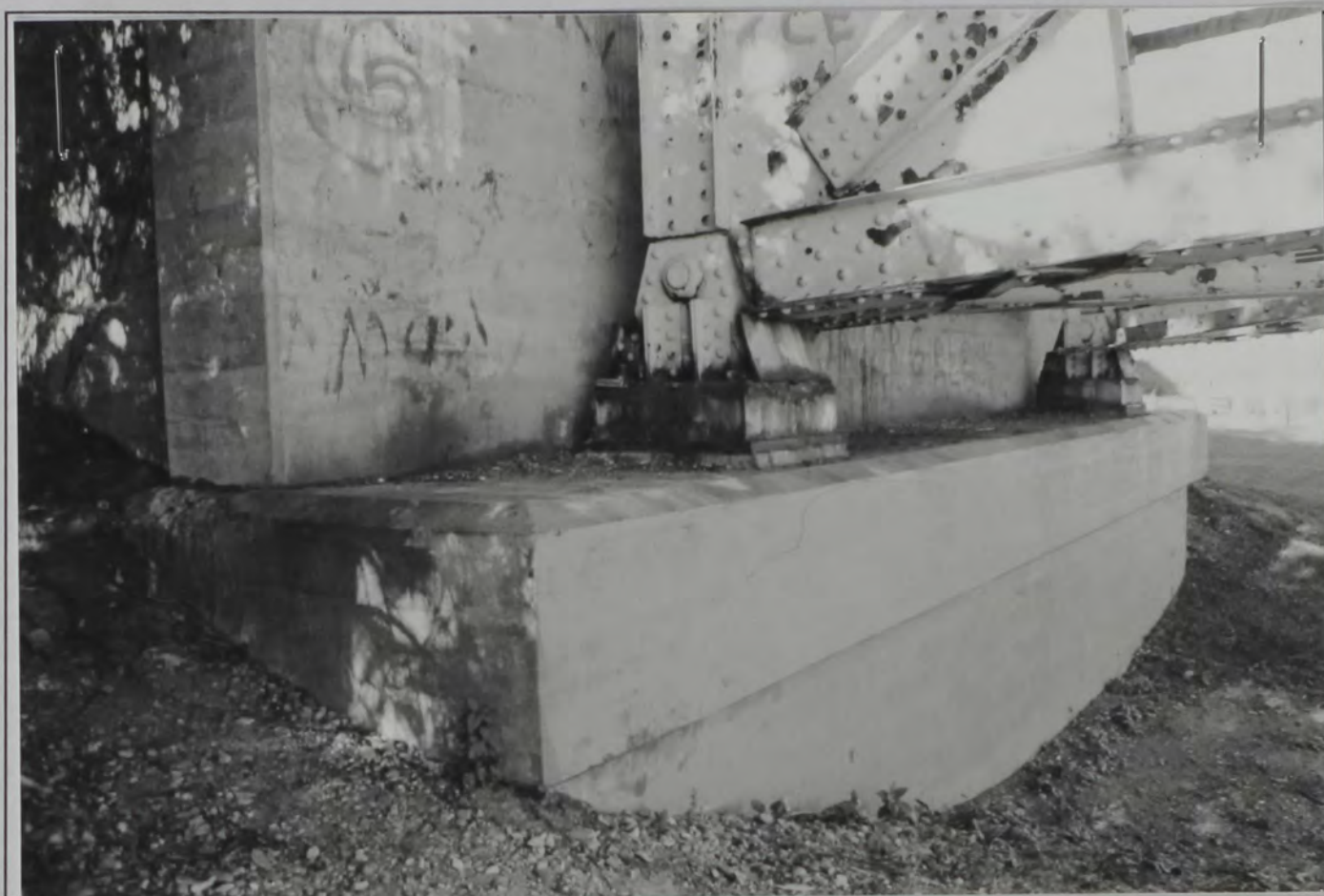
Photo 14: Detail of Rocker Bearing
